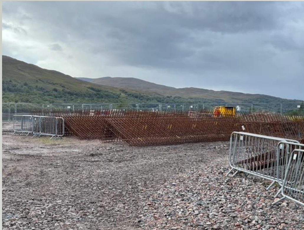
Progress Photos – Rebar fabrication at compound area.
