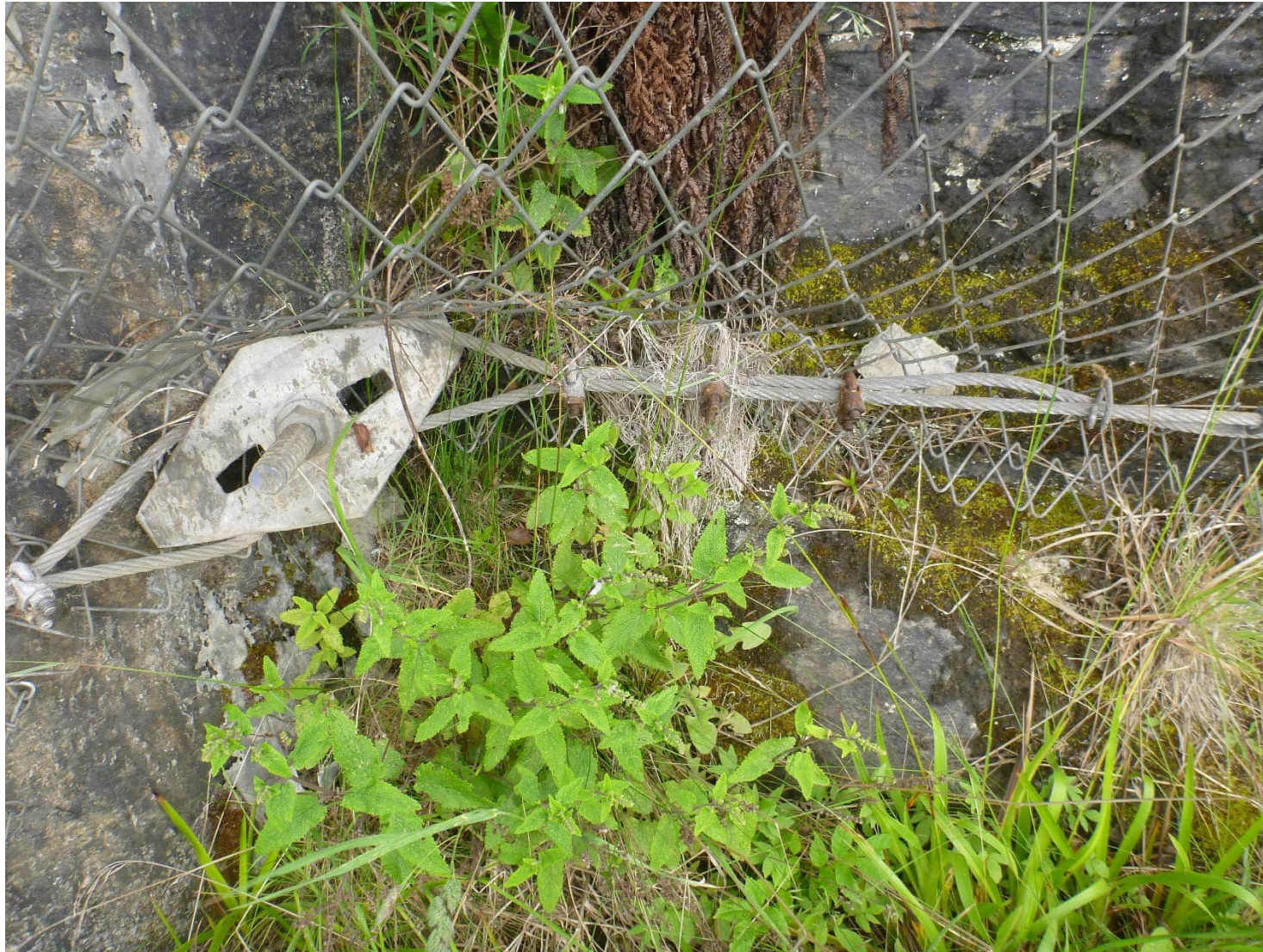
Example of some of the cable clamps on the bottom cable are starting to corrode at Ch. 3100.
