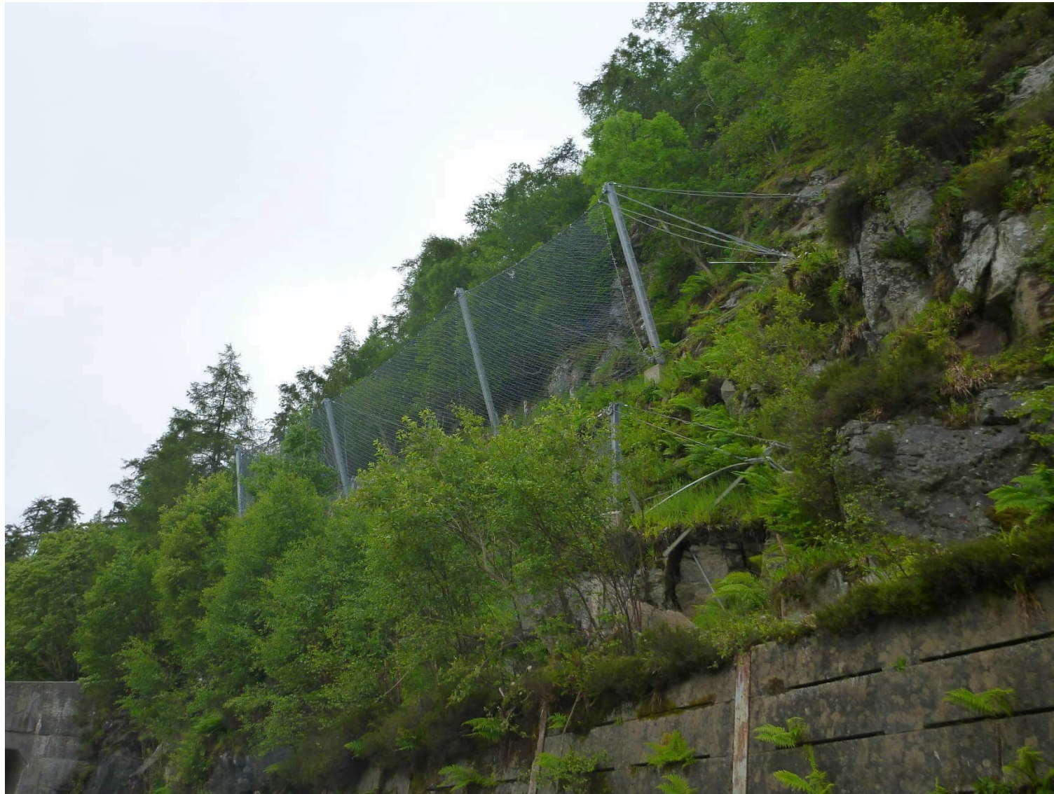
Catch fence installed during the Phase 12 2021 works
