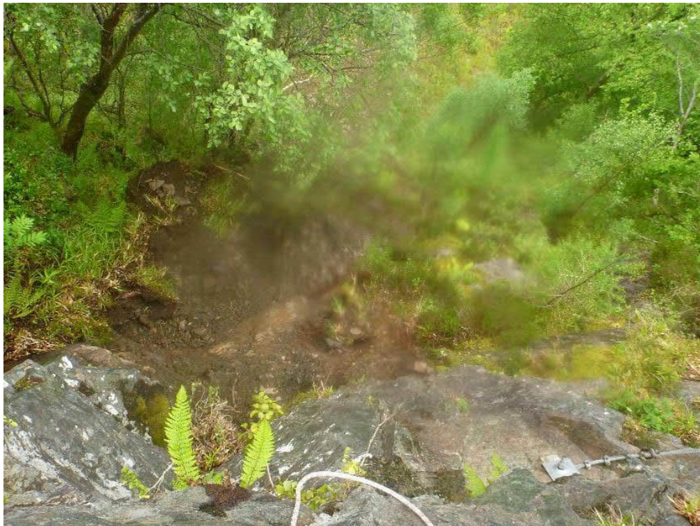
Photo 9: View downslope of failure source area from upper crags.
