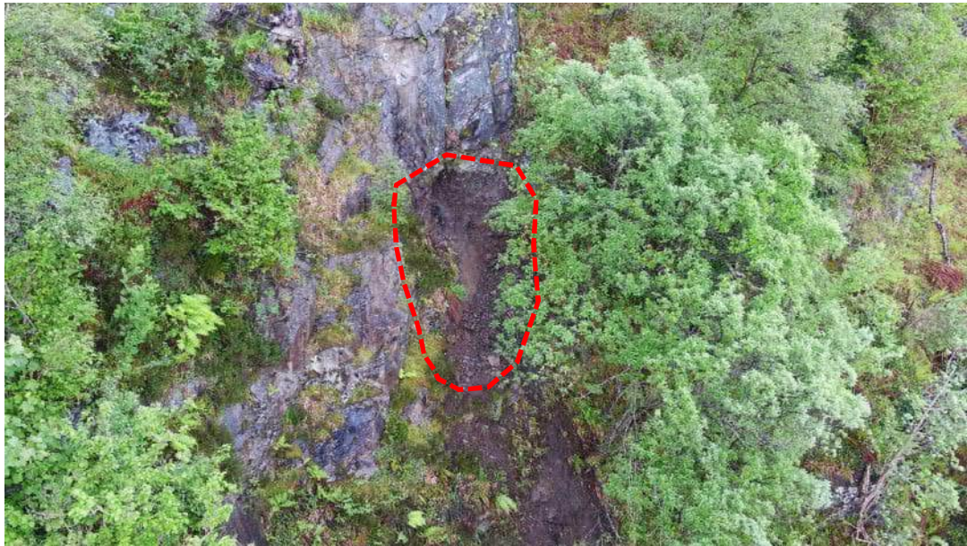
Photo 6: Failure source area circled.
