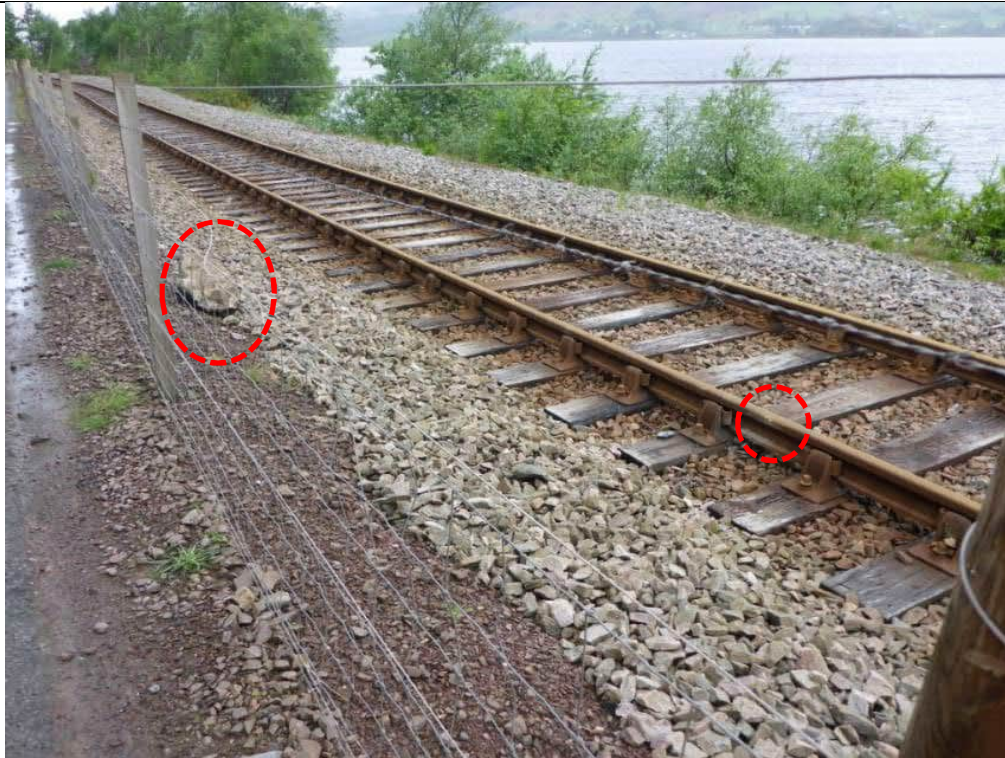
Photo 4: Block located in railway cess is highlighted above. Broken fence wire indicates it struck fence at ca. 0.7m height. Location of small impact mark on rail line also shown.
