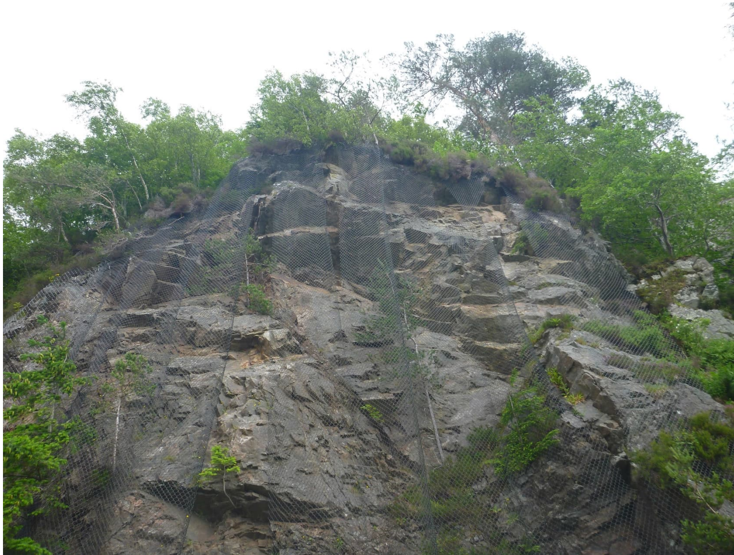
General photo of hazardous area at rock slope including the large overhang c.3 to 5m below crest of slope.
