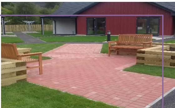
• Hilton Primary School, Exterior Nursery Unit
