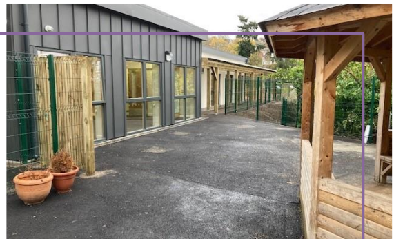
• Avoch Primary, Exterior Nursery Unit
