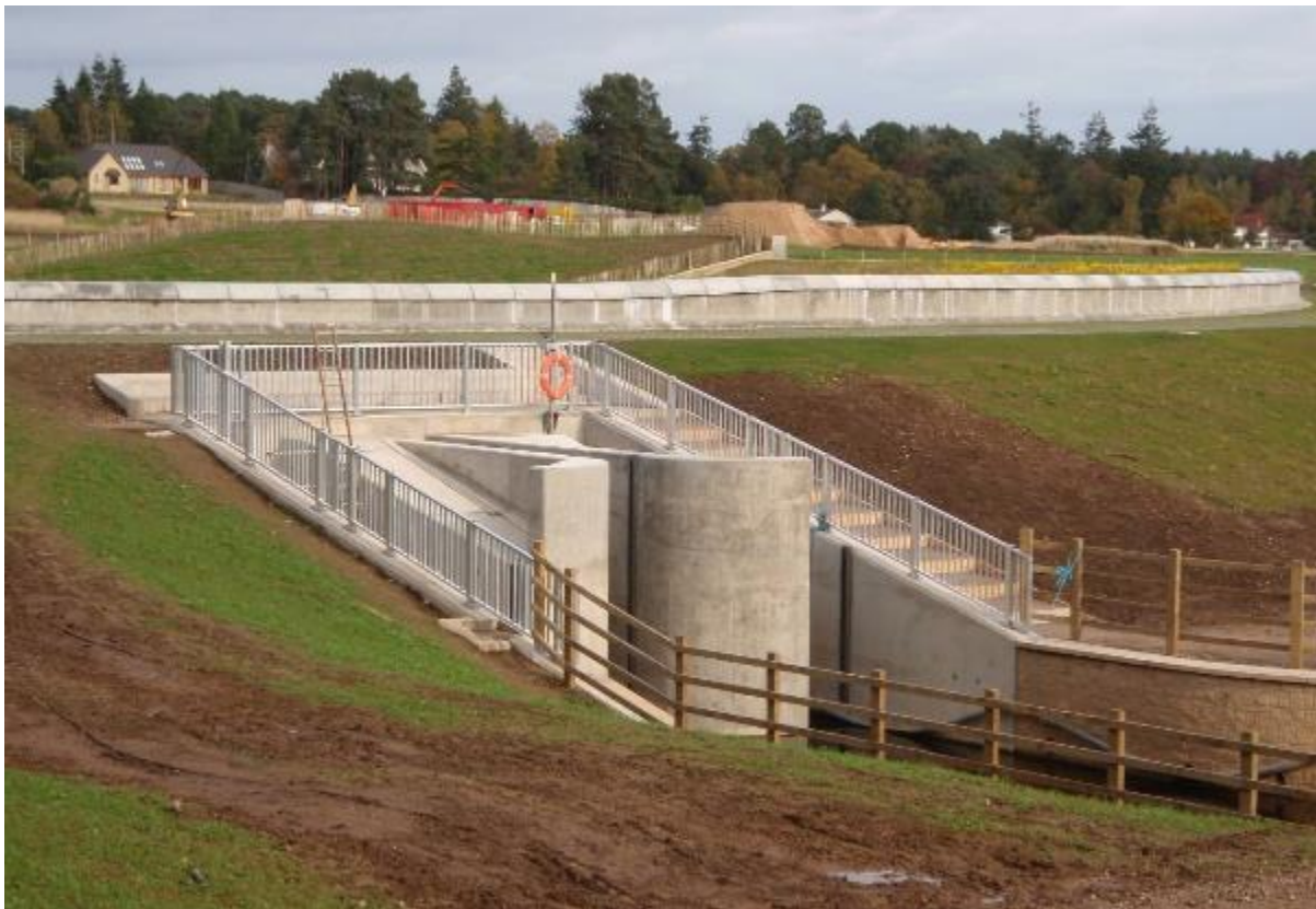
Chapelton Flood Storage Reservoir.
