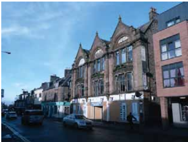
A. I. Welders and The Phoenix, Academy Street.
