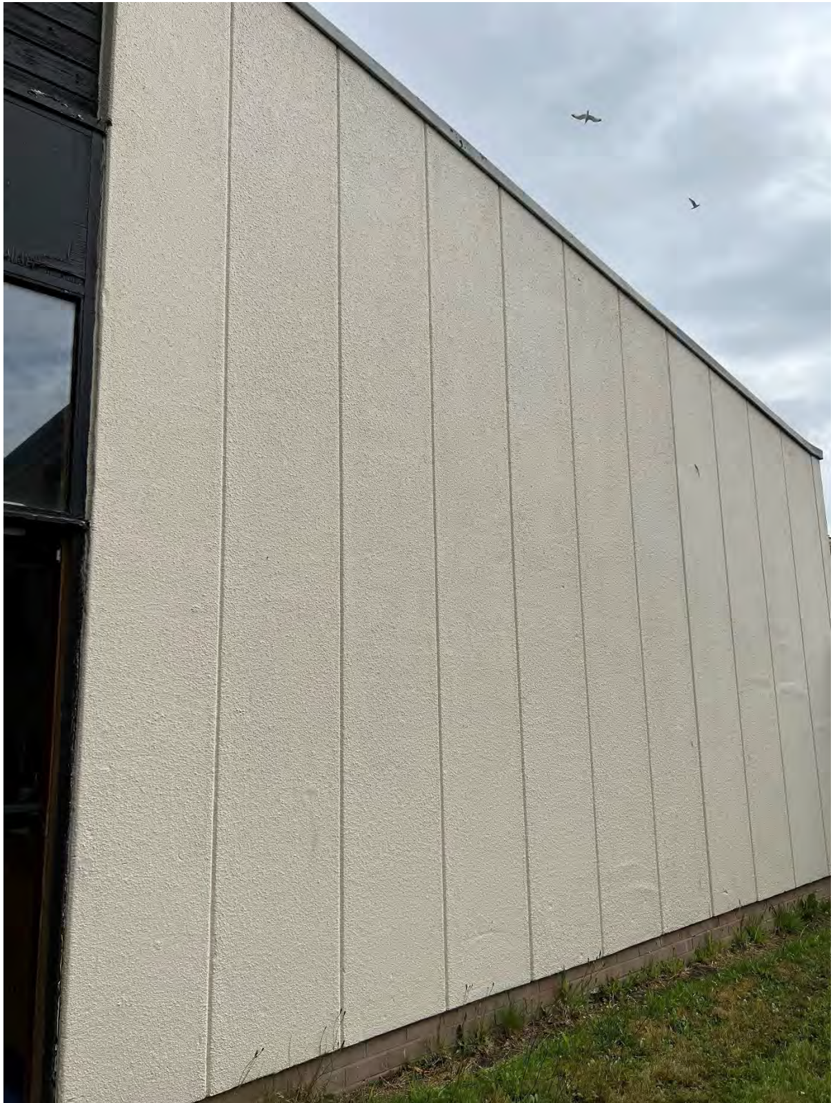
Photo N.8 – External view of Siporex Wall panels (Art Dept)
