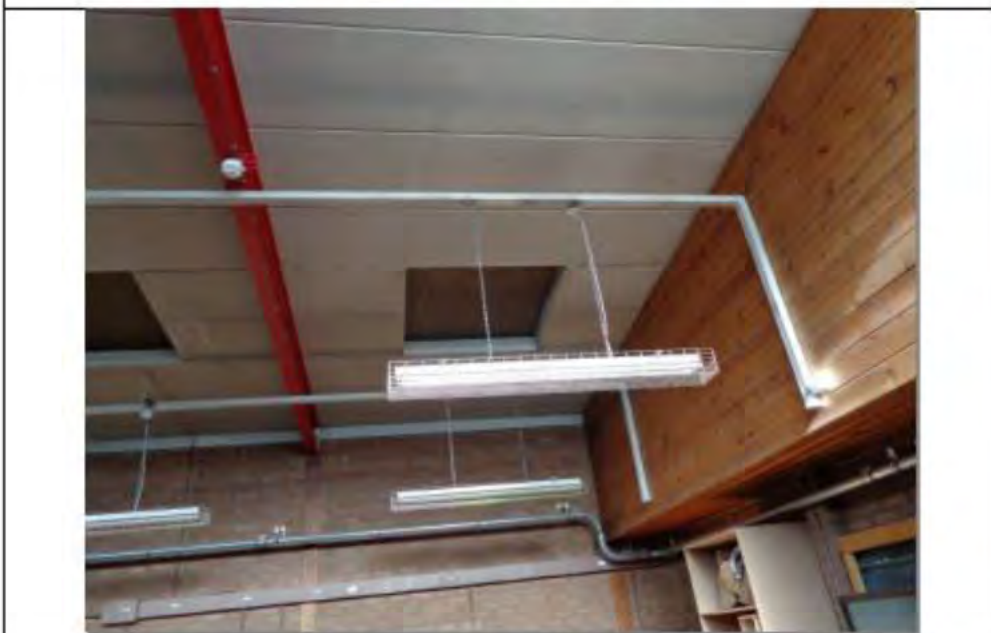
Photo No 2 – Typical view of the underside of exposed Siporex panels
