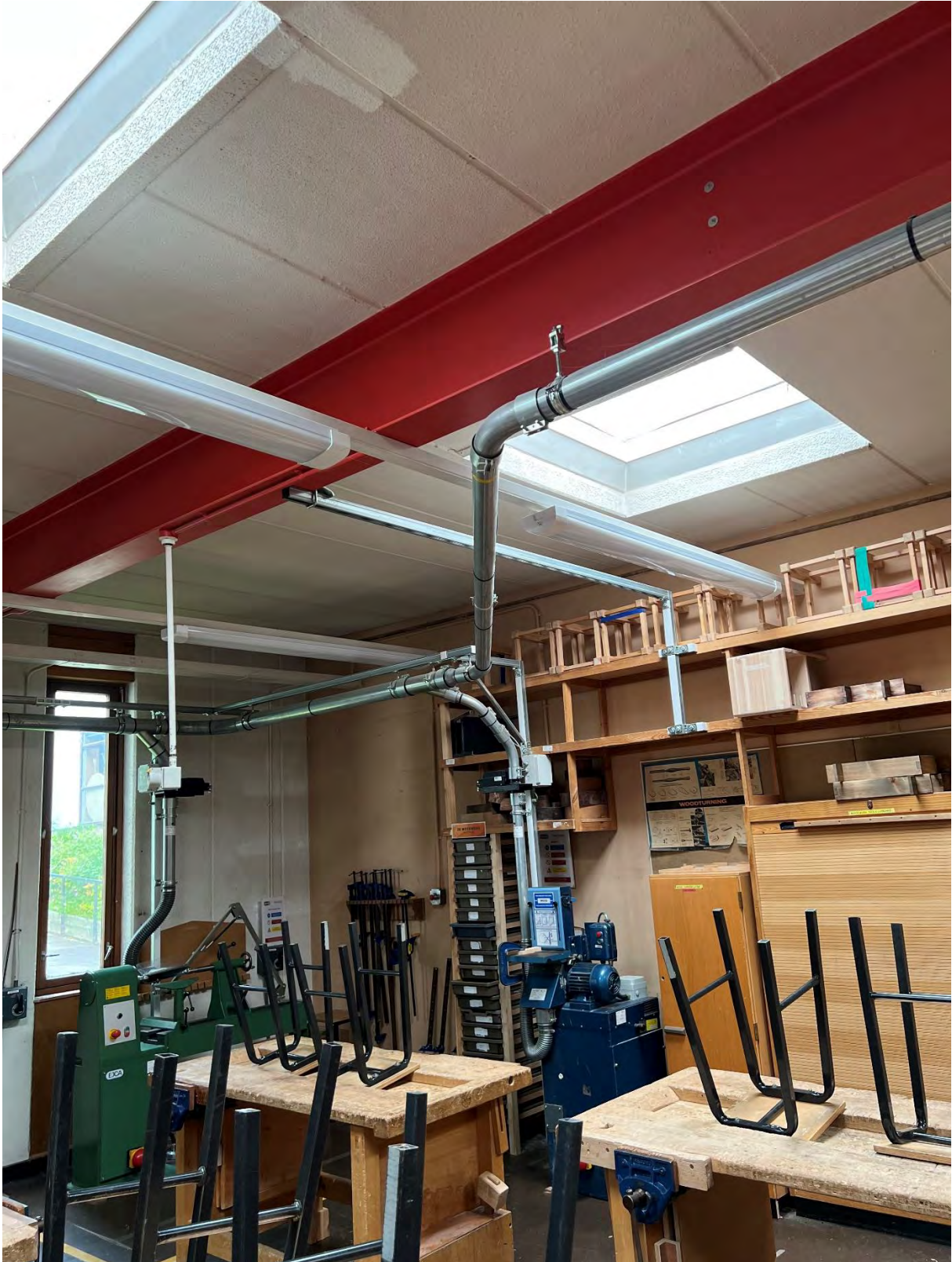
Photo N.1 - Bearing length appears to be less than 75mm throughout (Tech Dept)
