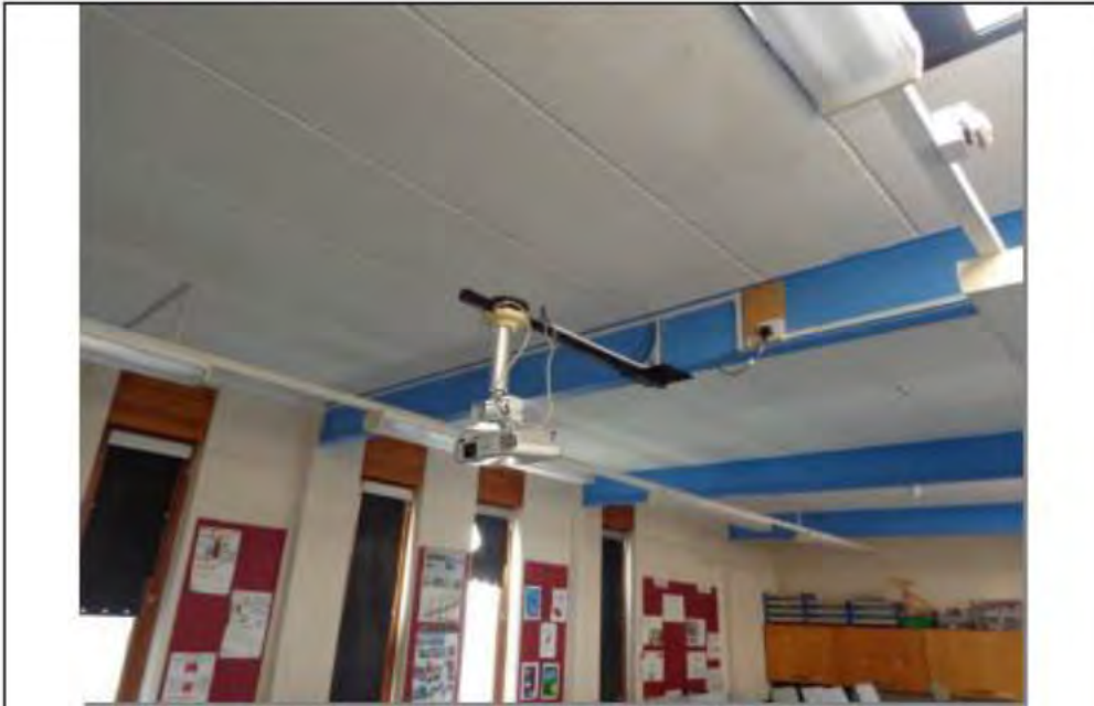
Photo No 1 – Typical view of the underside of exposed Siporex panels
