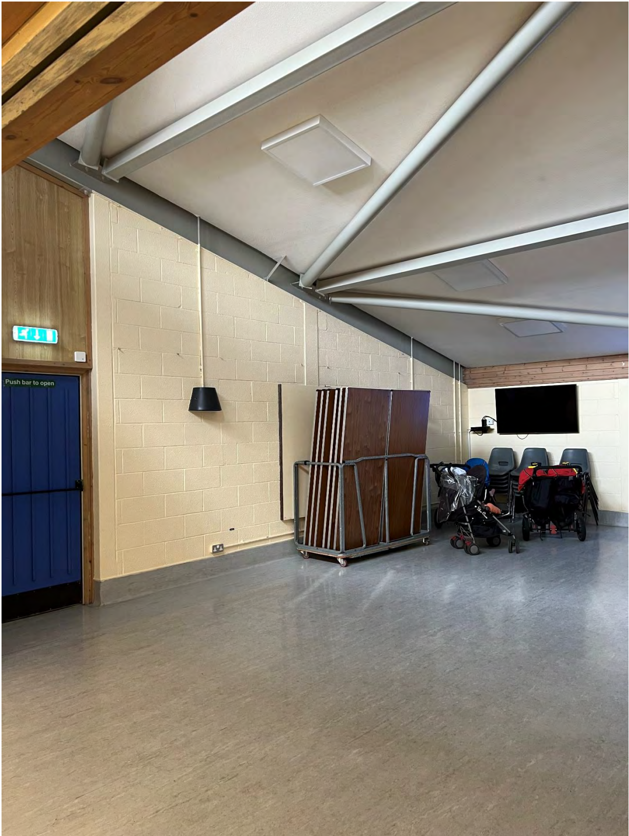
Photo N.21 – Newer Front extension constructed as steel framed (Community/gym block)
