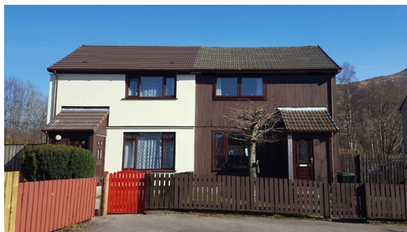
House on the left shows External Wall Insulation (EWI). House on the right shows house without EWI. Photos by The Highland Council.
