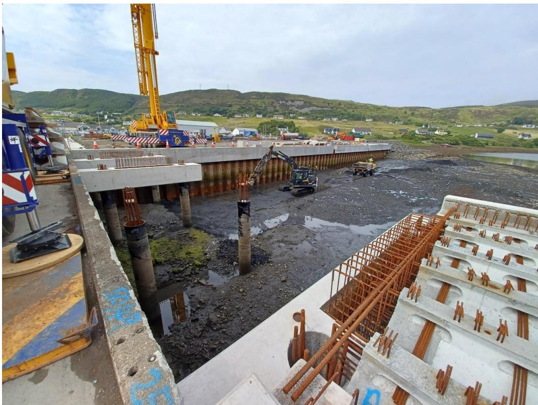
Dry Berth Excavation Works
