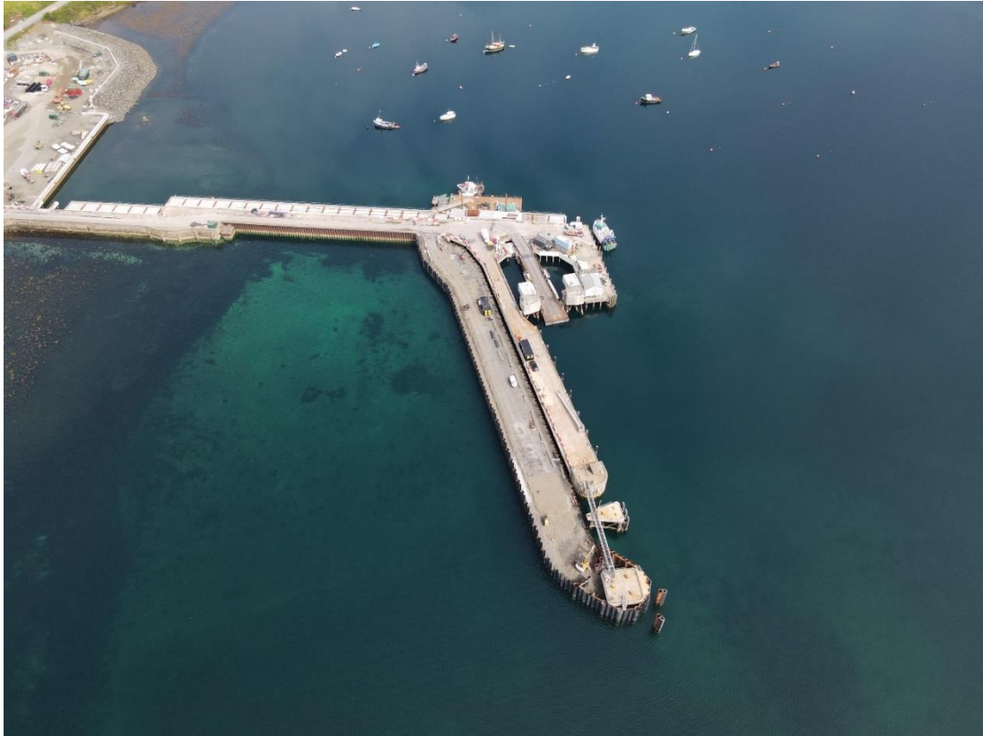
Berthing Structure Widening – Completion of Piling
