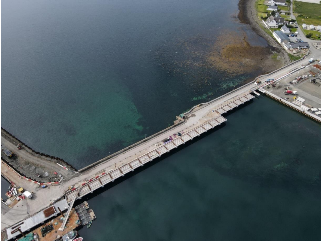
Approachway Widening – Installation of Precast and Concrete
