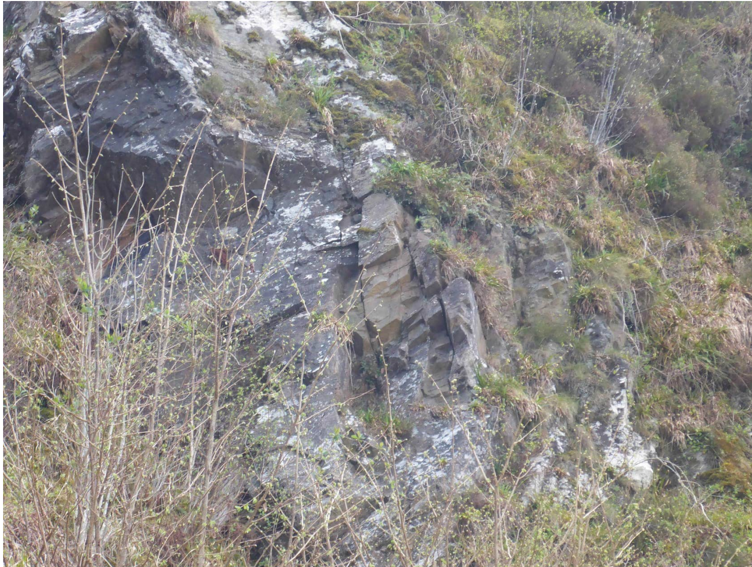
At Ch. 1803 - Dilated fractures observed c. 15m above road level.
