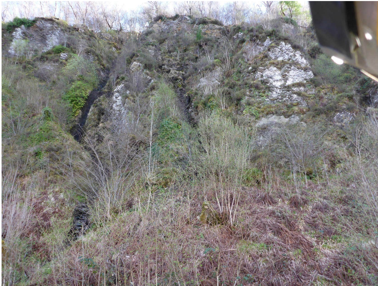
At Ch. 1820 - Fractured rock on right hand side of previous washout
