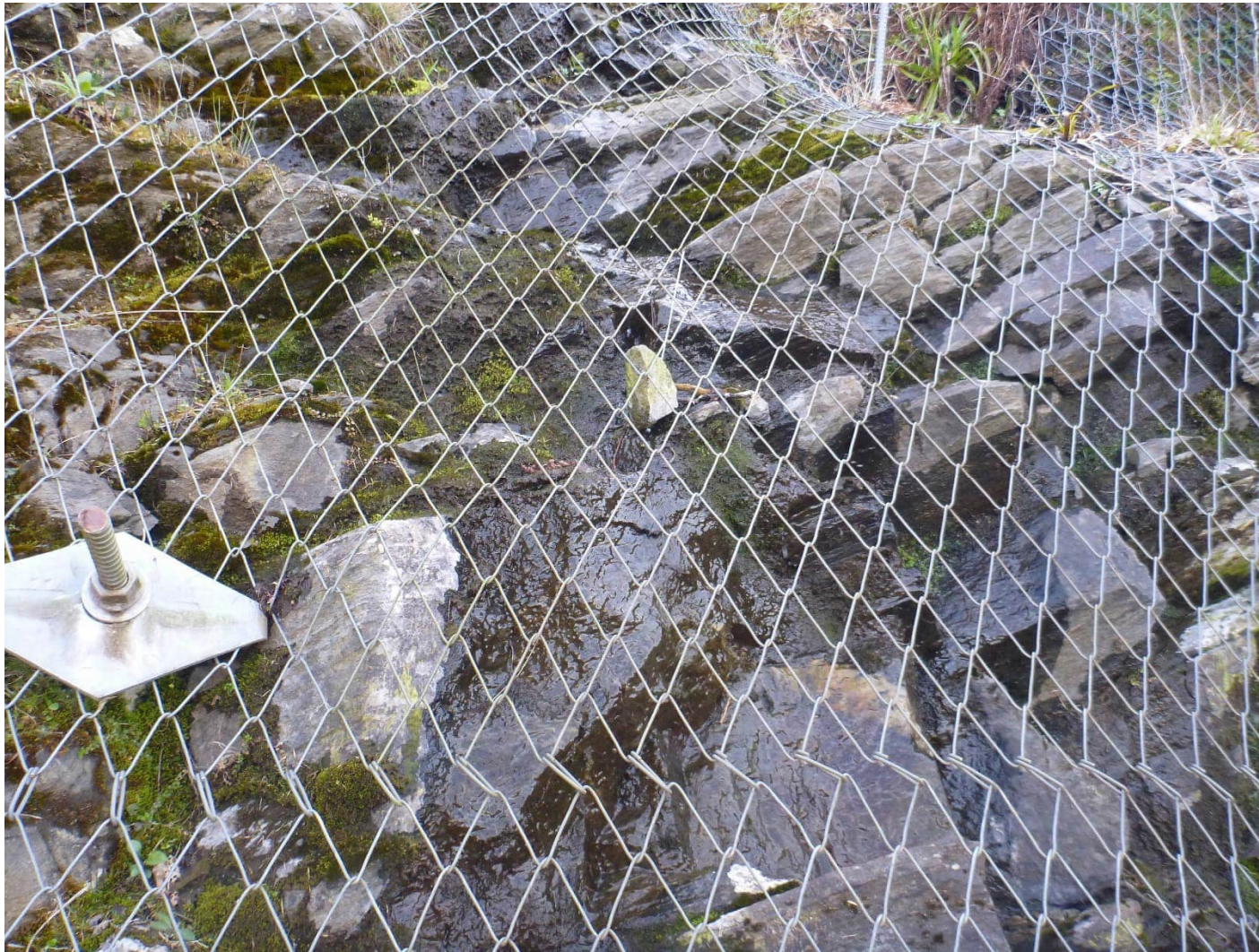
At Ch. 2990 (rope access) – TECCO netting in good condition
