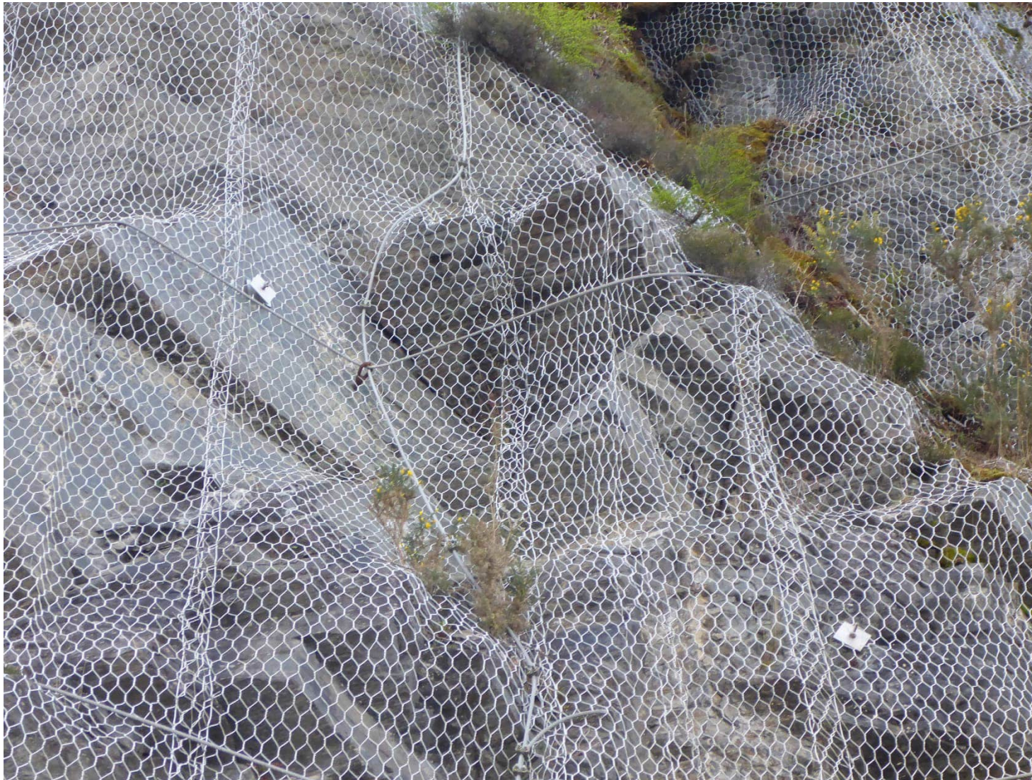
At Ch. 2965 - Large wedge approximately 10m above road level, with smaller wedge above.
