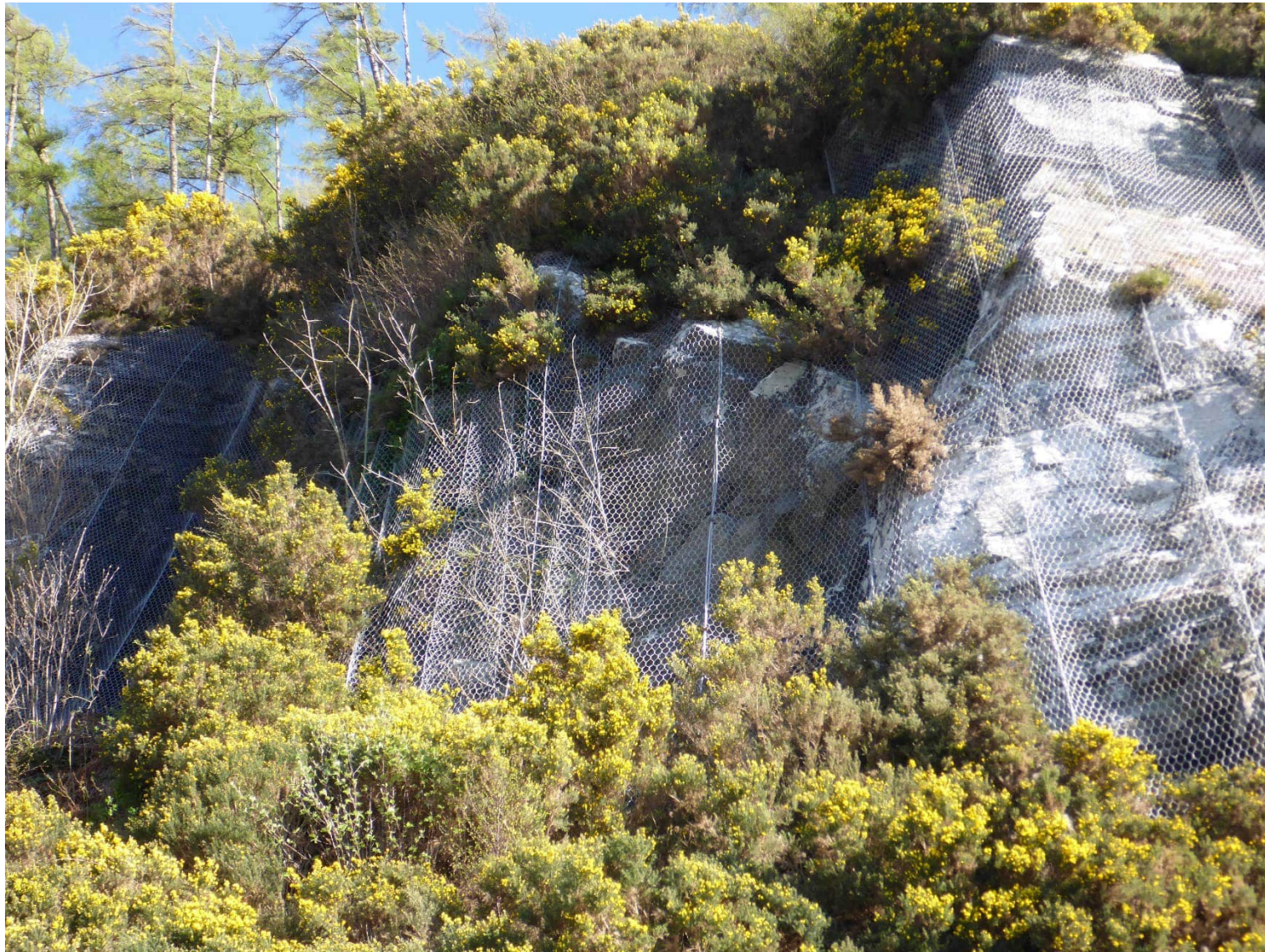
At Ch. 2535 - Overhanging area c.12 to 15m above toe with gapping mesh below
