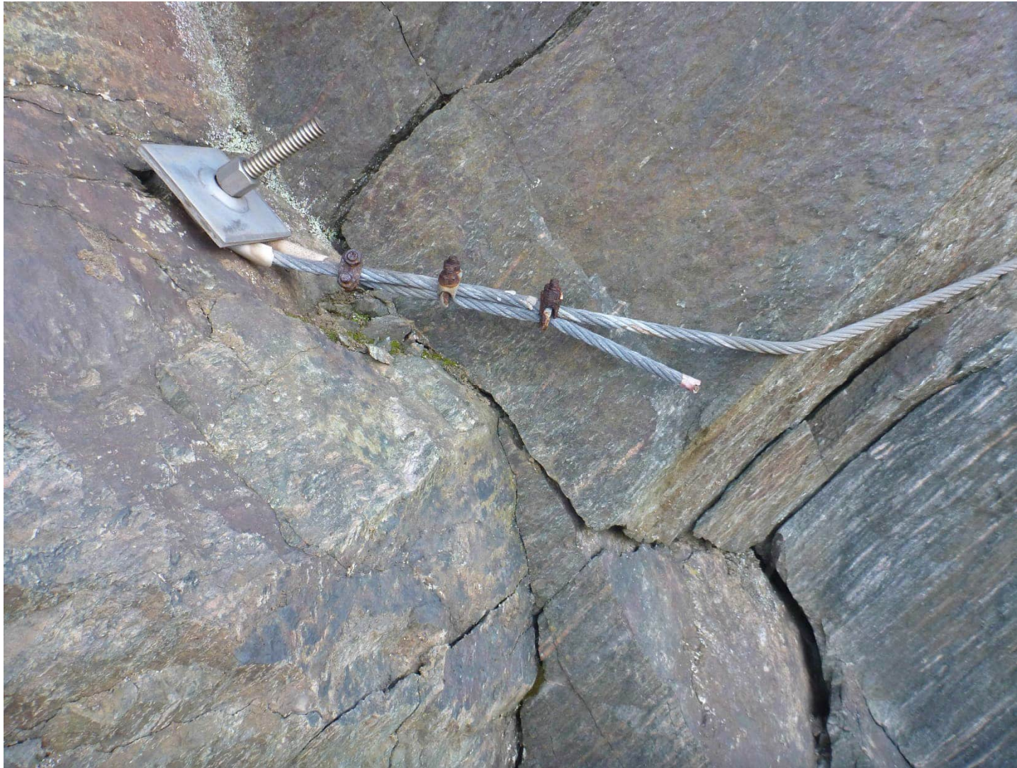
At Ch. 3350 (Rope access) – Cable clamps on cable restraint are corroded
