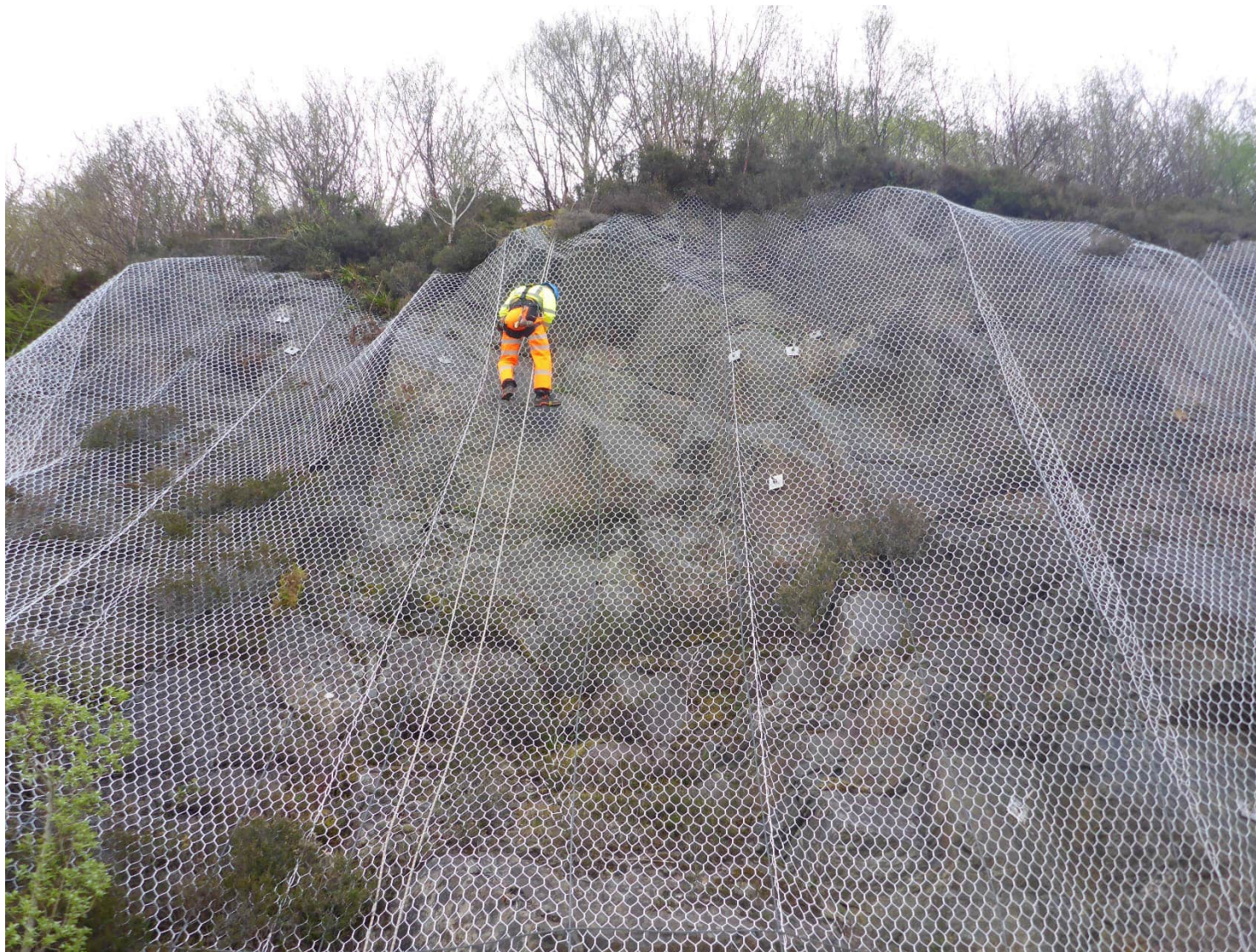
At Ch. 3350 - Rope access inspection undertaken to inspect area of overhanging/fractured block.
