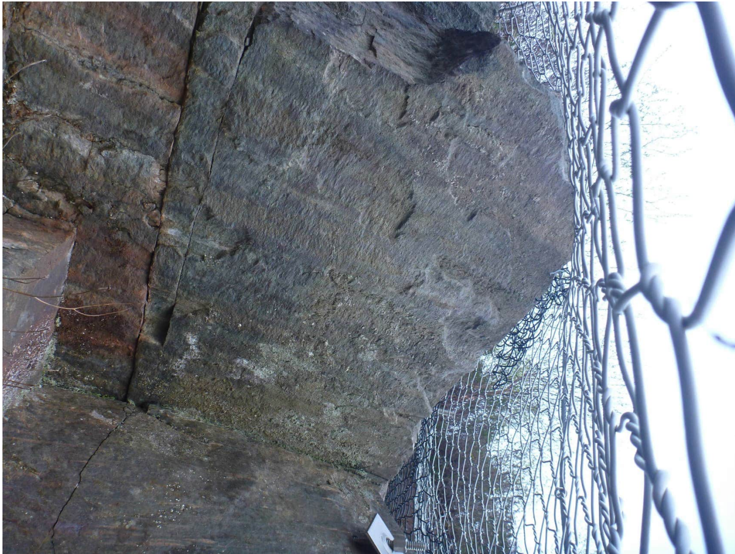
At Ch. 3350 (Rope access) – Overhanging rock mass ca. 1.5m and gape below is 2m
