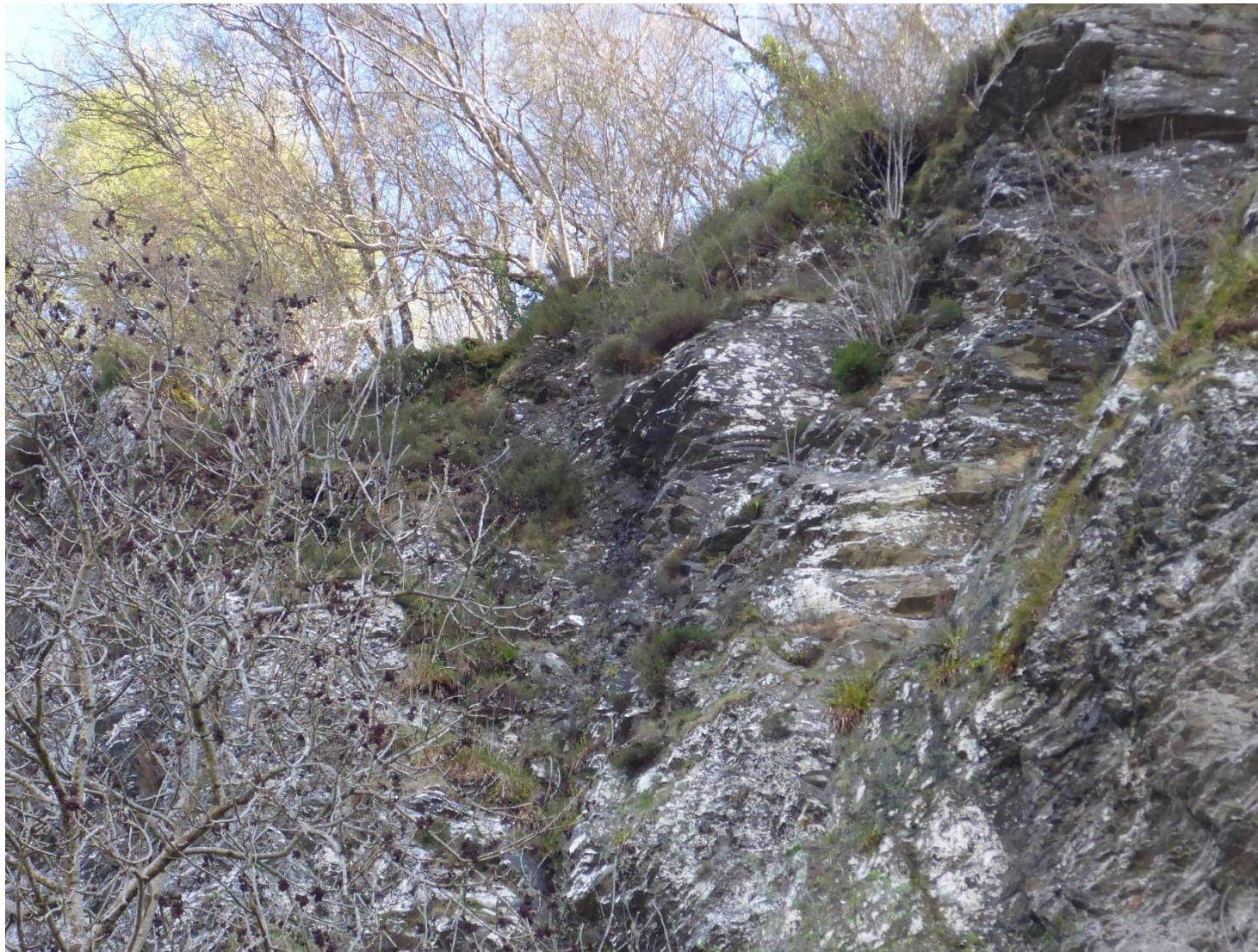
At Ch. 2000 - Large scale potential wedge failure. Is c.10m wide x 10m high feature at the crest of the rock slope
