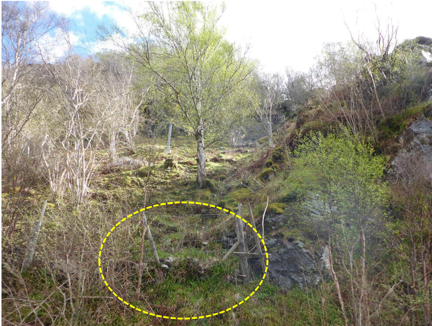
At Ch. 1505 - Accumulation of blocks at deer fence ca.3m above road level, along 5m length of slope.
