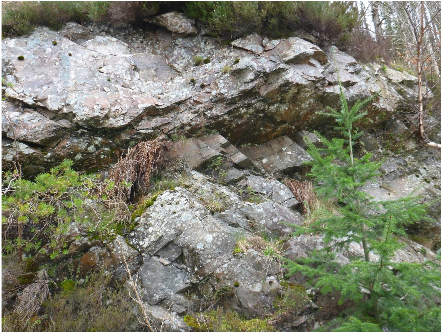
At Ch. 311 – Localised overhangs with potential for rock fall of unsupported blocks.
