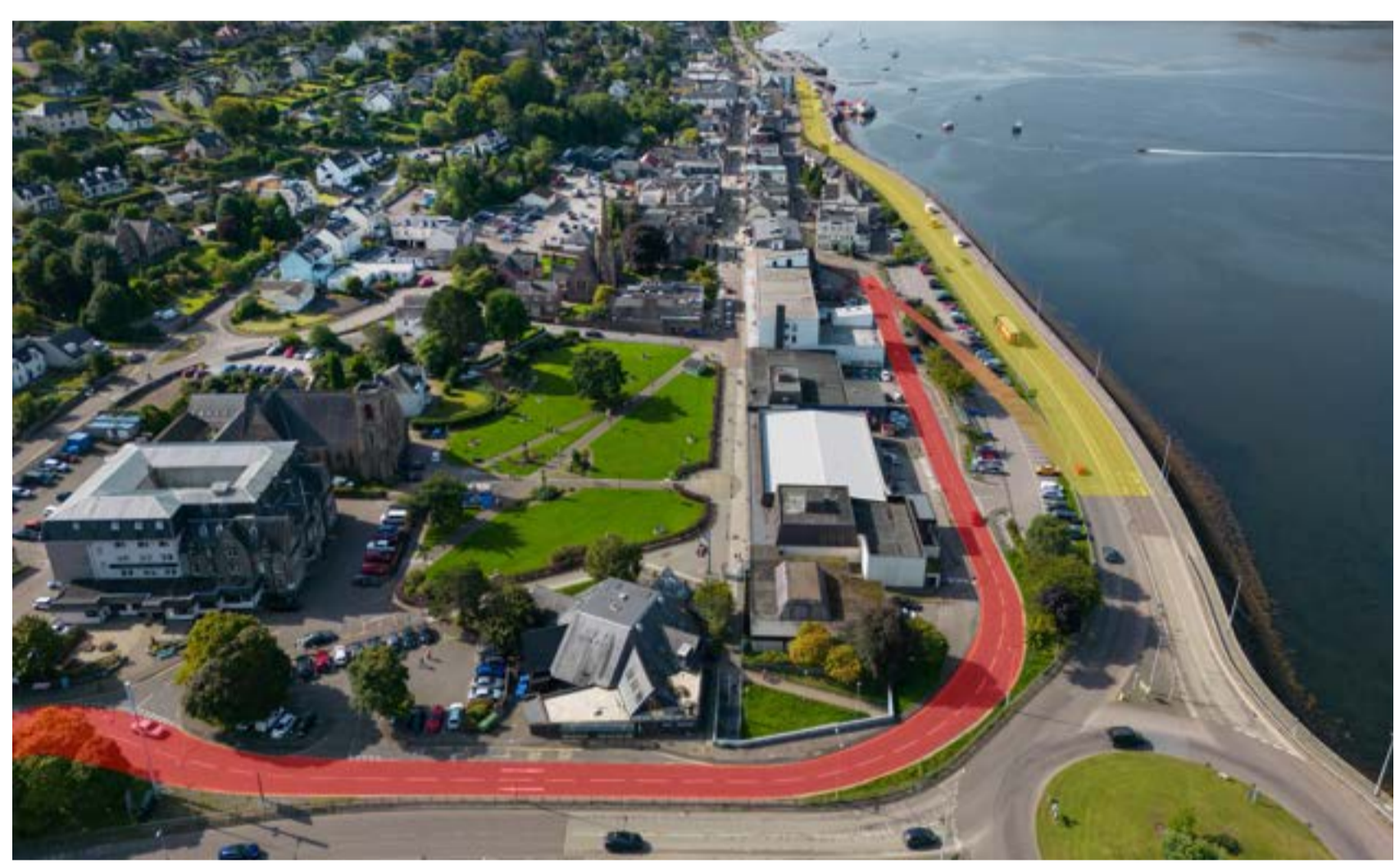
Removal of Middle Street A82 Reduced Lanes
