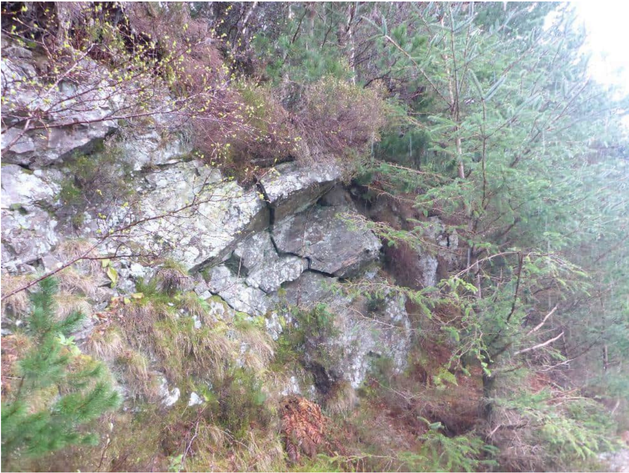
Photograph M1-1 Ch. 020 – block (c.2m x 1m x 1.5m) with dilated back fracture (poses low risk to road due to presence of verge). Year observation first noted: 2022
