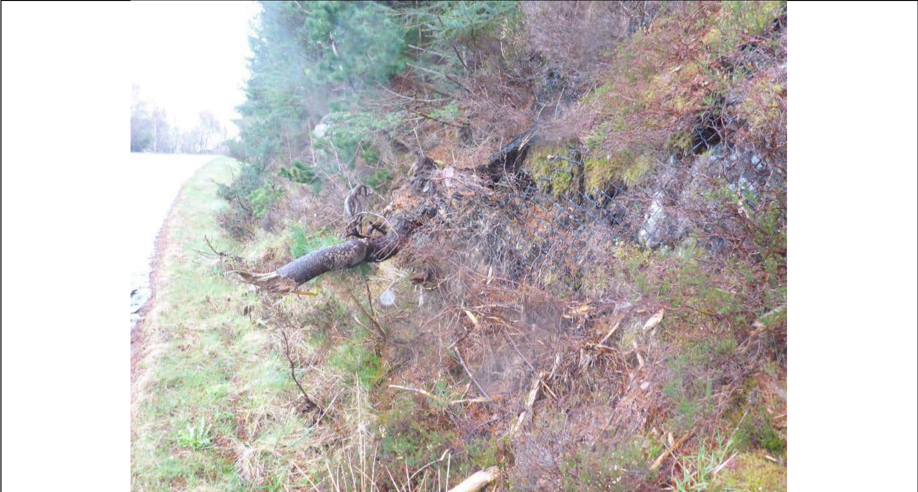
Photograph M1-2 Ch. 032– Rotated tree root protruding from rock slope. Year observation first noted: 2024
