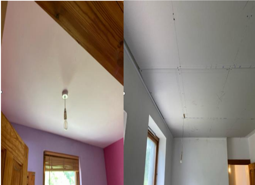
Figure 5 – Before and after install of IWI prior to taping and painting
