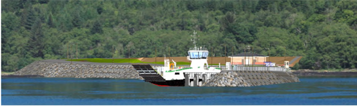
Figure A.5: Proposed Nether Lochaber Breakwater with Fendered Vessel Alignment Structure
