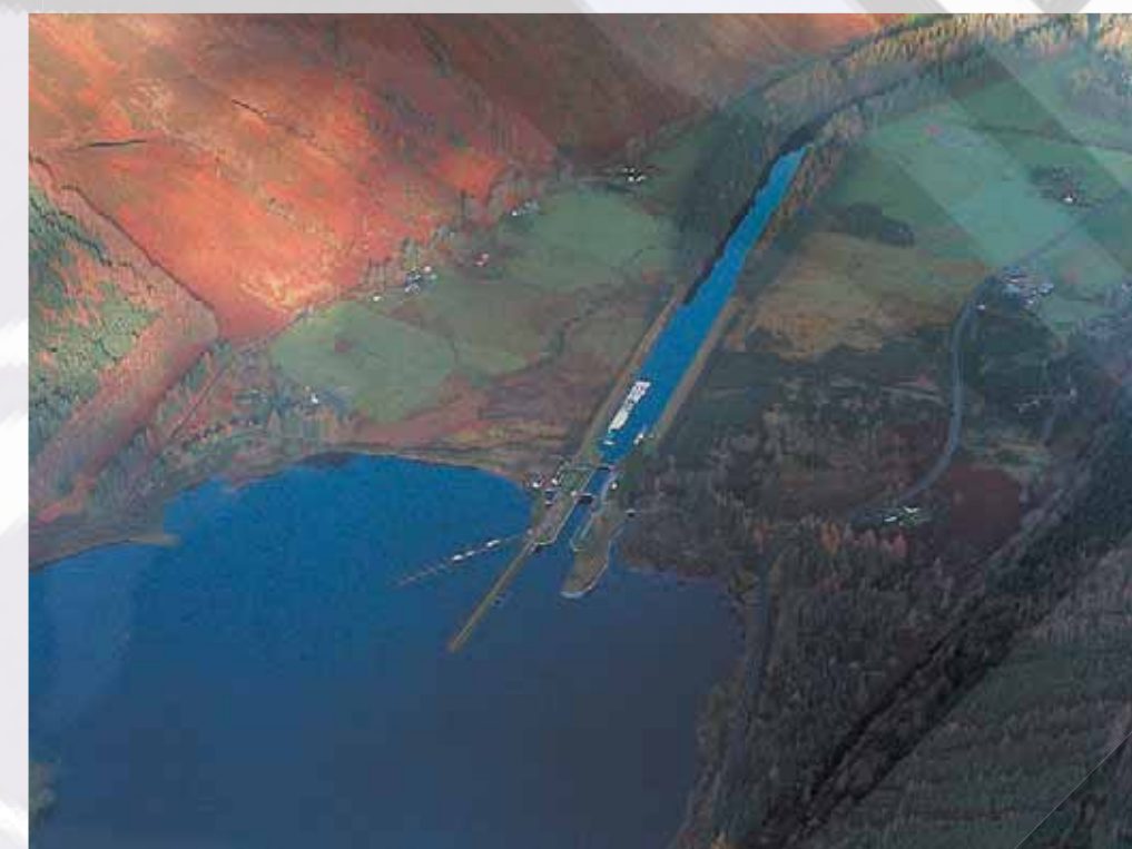
Aerial view of Laggan Locks.
