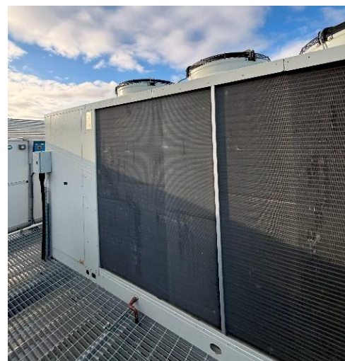
Figure 3-3: LSIC ASHP plant
