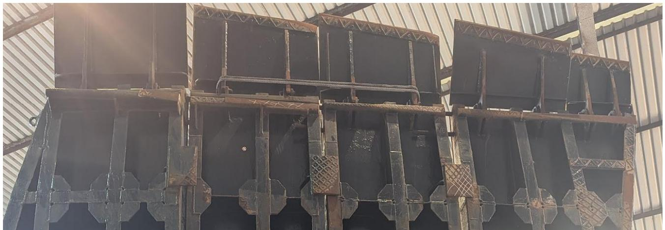
Existing stool structure and grounding bars have clearly been subject to multiple rebuild & additions in the past, to the extent that further localised repair or rebuild is considered to be neither practical nor a cost effective solution. As a consequence rebuild of the stool structure to include replacement of all sacrificial grounding bars is recommended.
