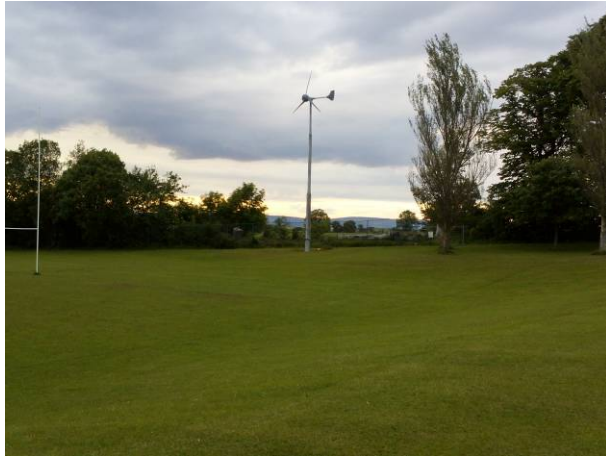
Figure L6-view of the turbine from the South
