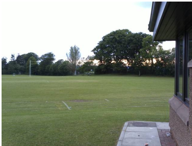
Figure L7-view of the turbine from the closest part of the school.
