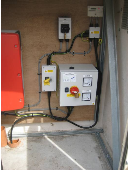
Figure J11-wind turbine controller and local distribution board (note: a temporary seal to the distribution board is made by electrical tape)
