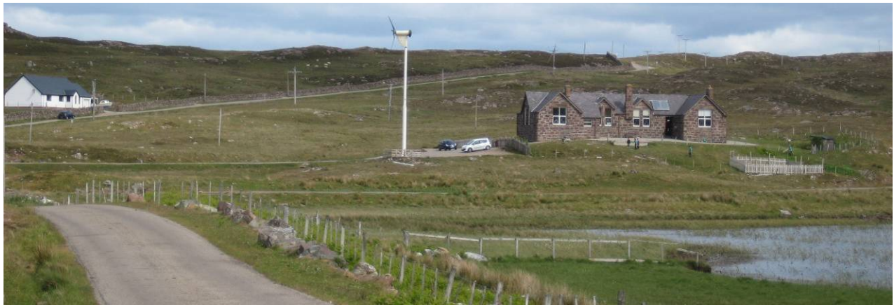
Figure J2-view of the site from the South
