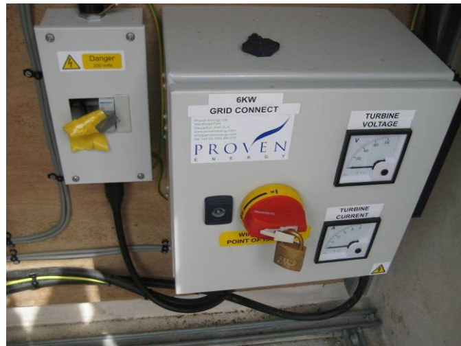
Figure J11-wind turbine controller and local distribution board (note: a temporary seal to the distribution board is made by electrical tape)
