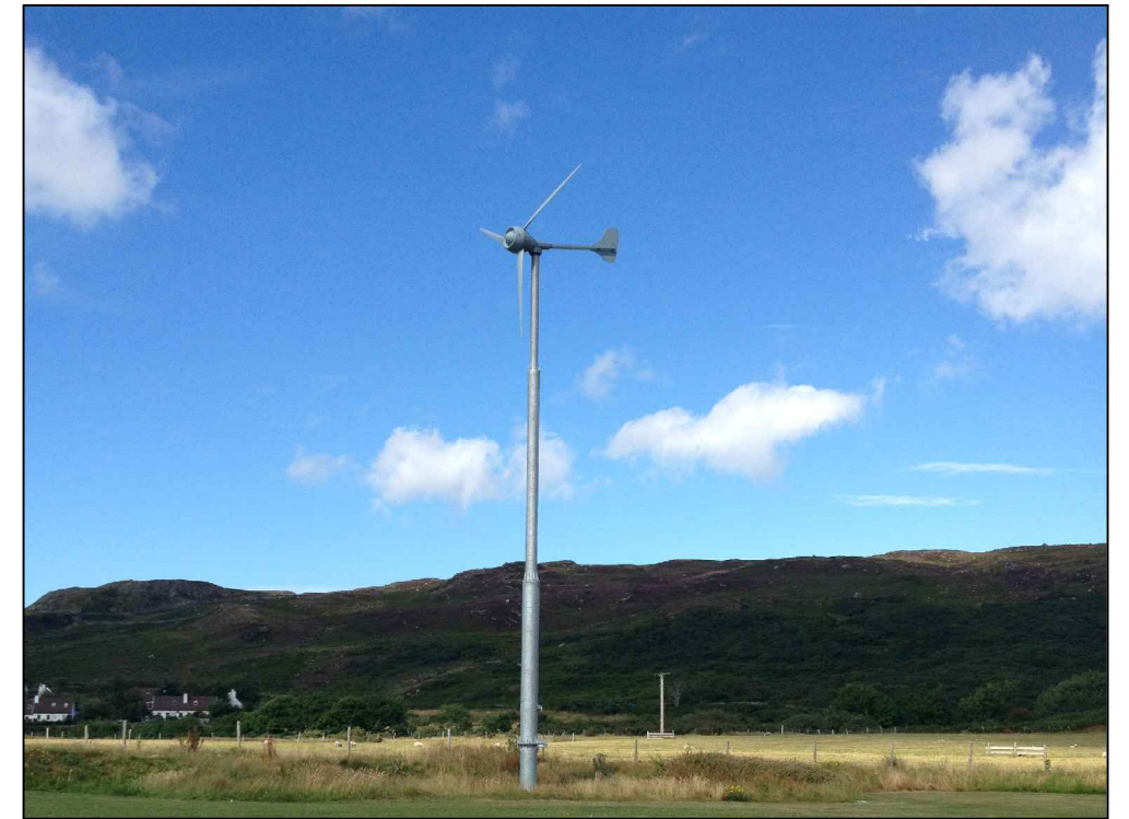
View of Turbine from School Building
