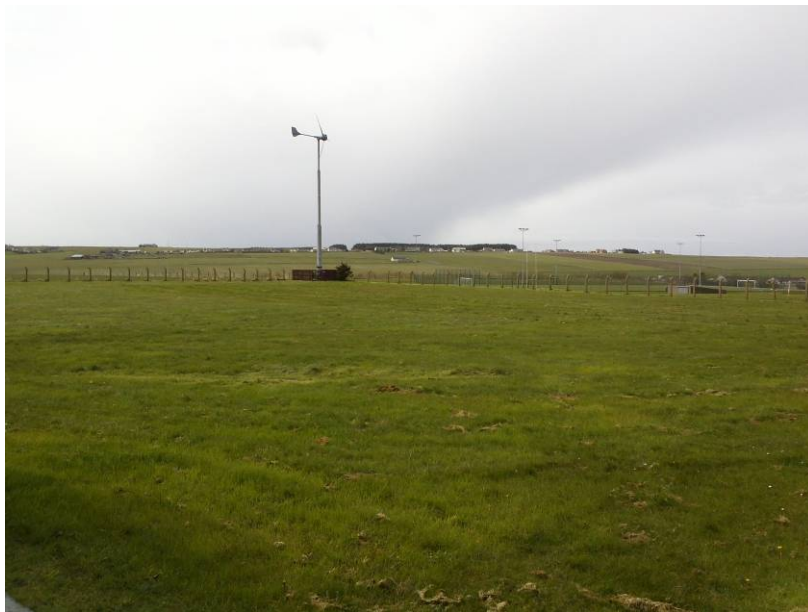
Figure E6-view to the turbine from the closest point of the school building
