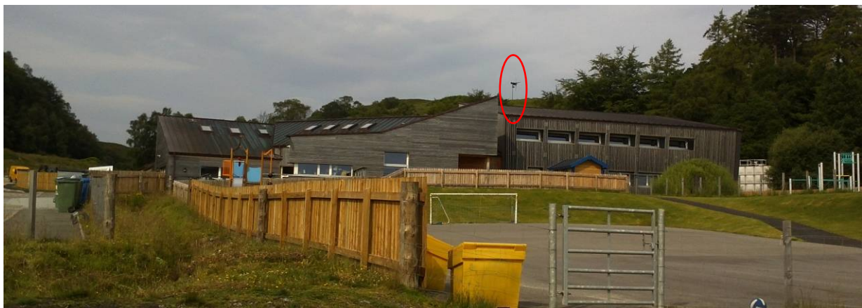
Figure M10-view from the school access road to the West
