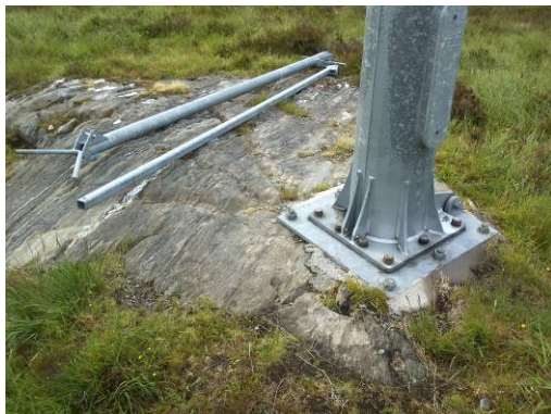
Figure M3-rock-anchor base
