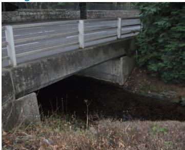
Figure 5.1: Culcabock Road Bridge
