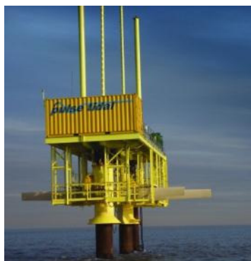
Figure 5 Pulse Stream 100 (0.1MW) TSD
