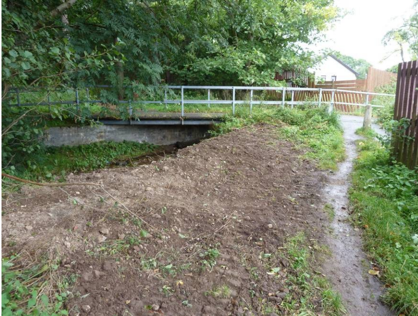
Figure 8-3: Repaired bank at location of bank overtopping into Smithton Villas
