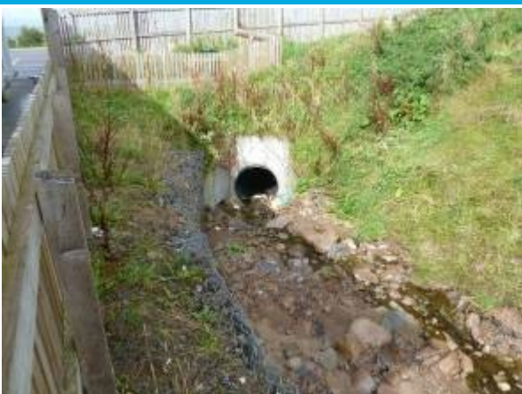
Upstream face of culvert
