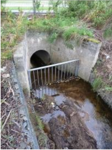
Upstream face of culvert
