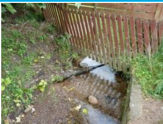
Downstream face of fence
