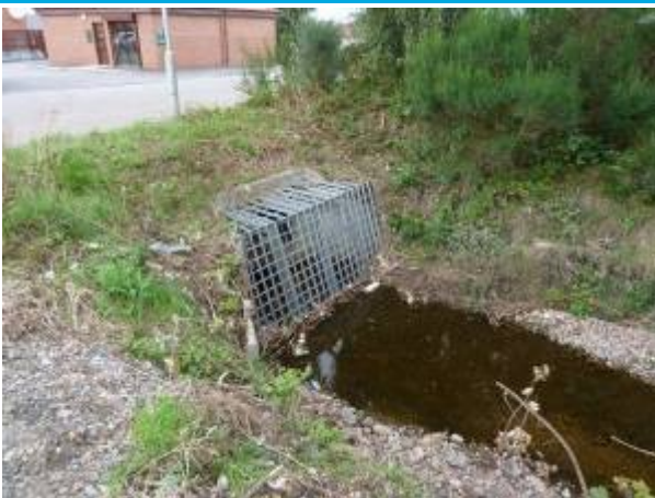
Upstream face of culvert
