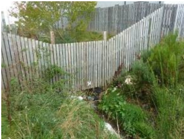
Upstream face of fence
