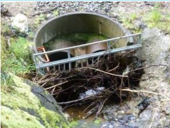
Upstream face of culvert
