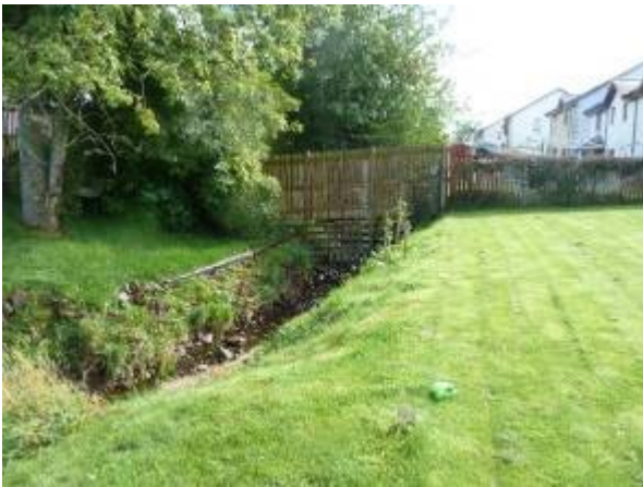
Downstream face of fence
