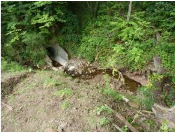
Upstream face of culvert
