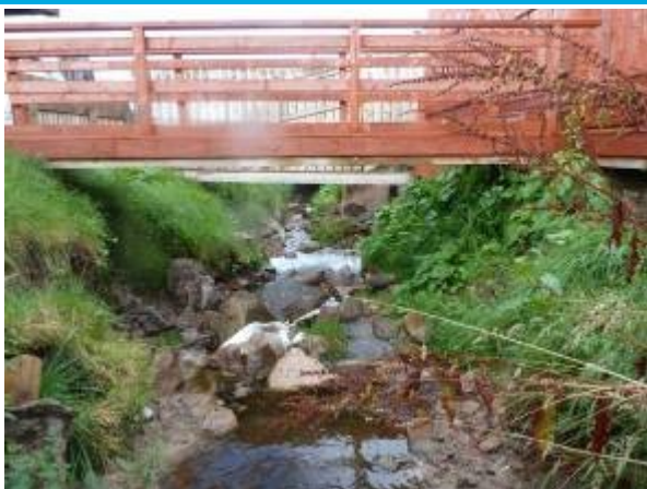
Upstream face of decking "bridge"
