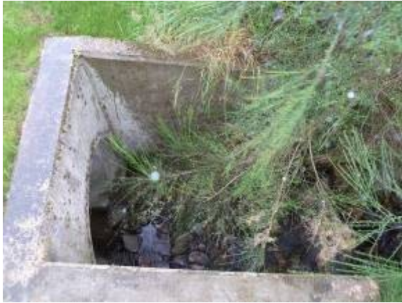
Upstream face of culvert
