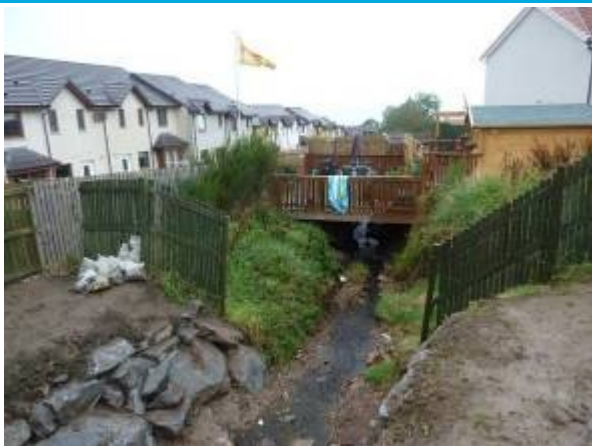
Upstream face of decking "bridge"
