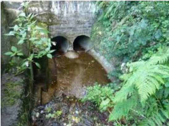
Upstream face of culvert
