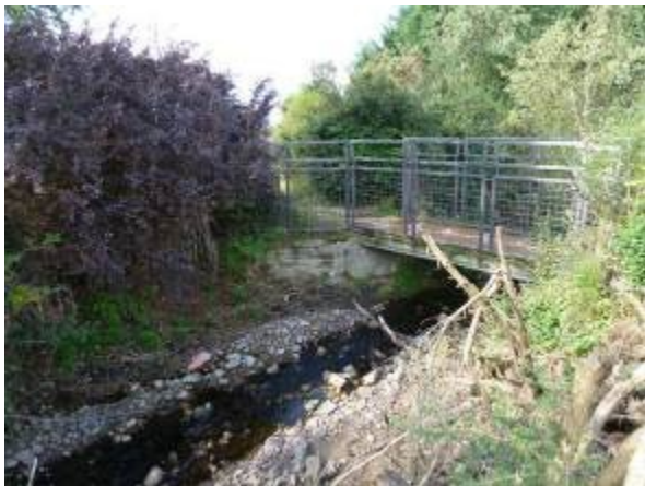
Upstream face of bridge
