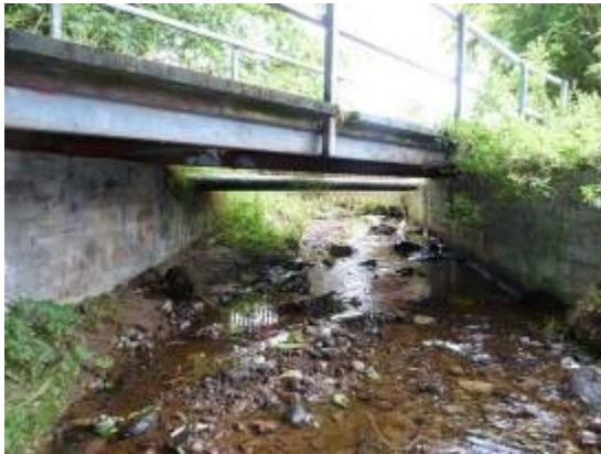
Downstream face of footbridge
