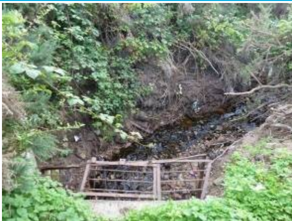
Upstream culvert inlet and channel
