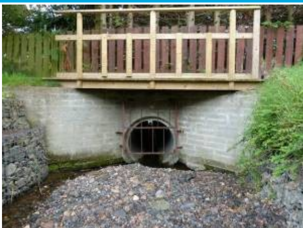
Upstream face of culvert
