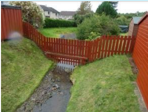
Upstream face of bridge
