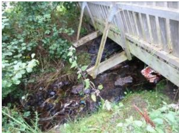
Downstream face of culvert
