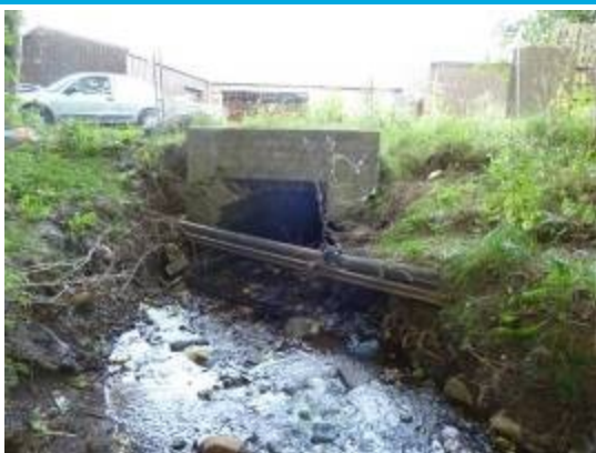
Upstream face of culvert
