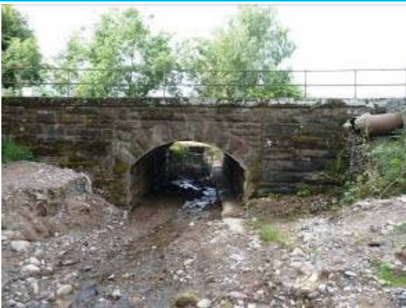
Upstream face of culvert
