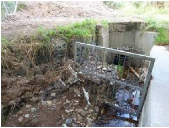
Downstream face of culvert
