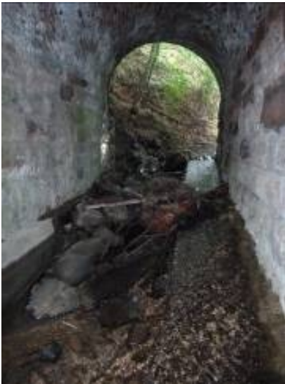
Upstream face of bridge
