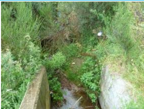
Channel upstream of culvert
