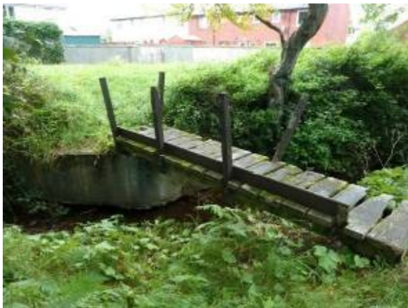
Upstream face of footbridge
