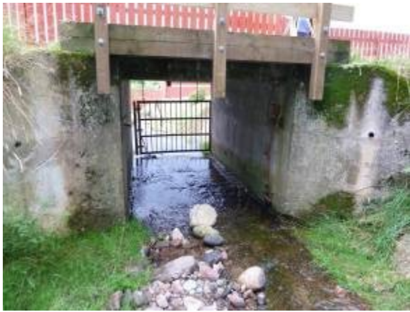
Upstream face of bridge
