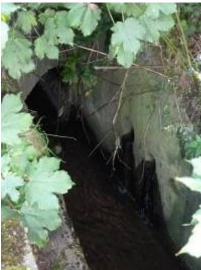
Upstream face of culvert
