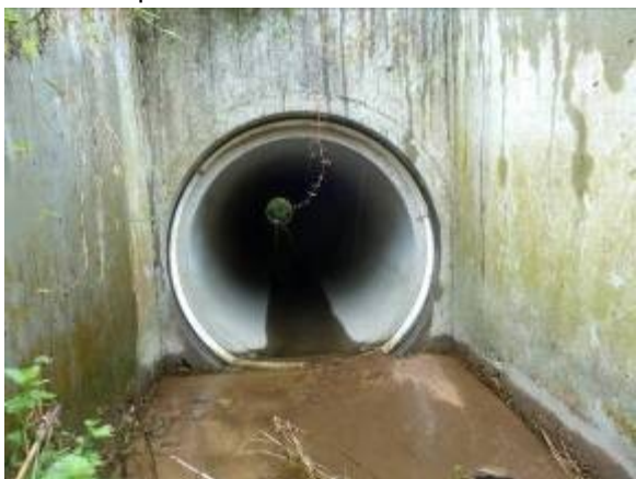
Upstream face of culvert
