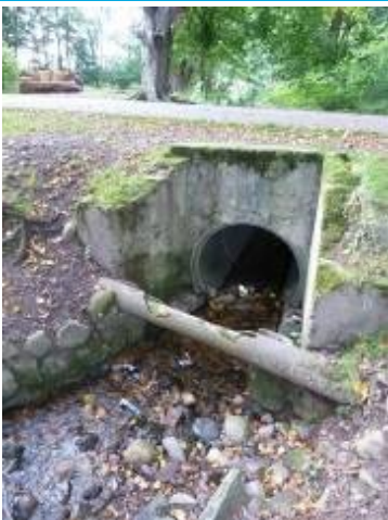
Upstream face of culvert
