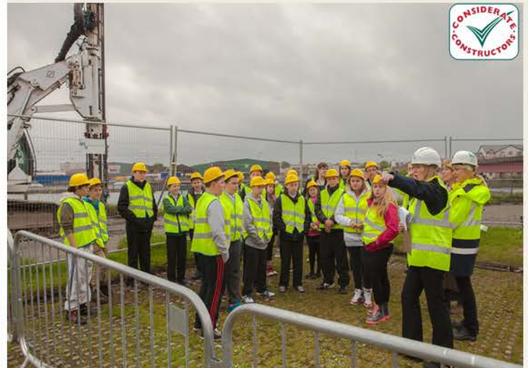
Image: Angela Ford, PR Liaison Officer for MCLH talking to the children from Merkinch Primary School, during their site visit. They were able to view the sheet piling machine whilst not in operation.
