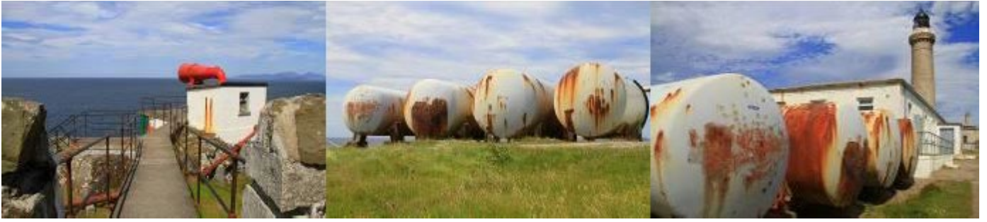
L to R: the foghorn viewing platform has huge potential to deliver safe pushchair and wheelchair access to a dramatic coastal landscape; accumulator tanks forming part of the foghorn mechanism; close-up of unsightly corrosion damage to these tanks, and the strong negative visual impact that their condition has on the site.
