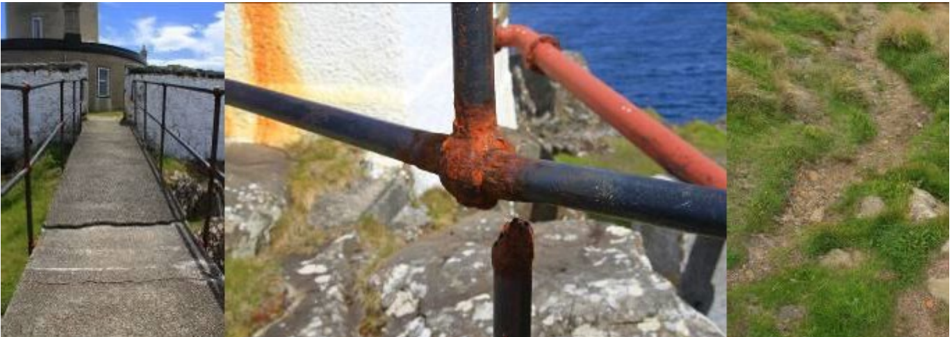
L to R: fractures in the walkway surface to the foghorn viewing platform (this area has huge potential to deliver safe pushchair and wheelchair access to a dramatic coastal landscape); close-up of the existing railings; example of an informal footpath on site, which we propose to upgrade to a level and durable finish.
