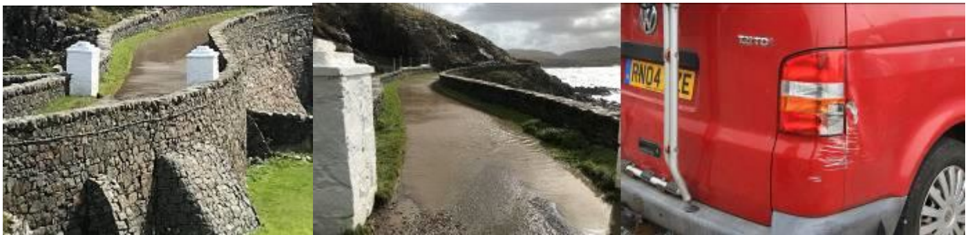
L to R: flooding on the causeway/central track resulting from poor drainage; this significant flooding restricts pedestrian/pushchair/cycle access and exacerbates erosion damage to the causeway/central track surface; damage caused to a campervan on the causeway in early July 2020, when an absence of traffic management required the driver to reverse (the walled causeway is 200m long, winding, and does not have passing places/room for vehicles to pass on the verge ).
