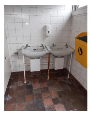
The bib tap has no cross head, if the plan is to use this for filling drinking water containers, I suggest fitting a percussion tap.
