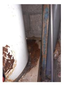
Toilets, the hand dryers in both toilets work but the casings are corroded and are unhygienic.
