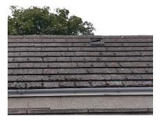
The roof verges are in very poor condition and are a health & safety concern for the public, the under cloak is cement board and this has been snapped off in places, all of the verge pointing needs to be replaced there are large areas missing and other areas that the pointing is hanging off of the top of the under cloak.
