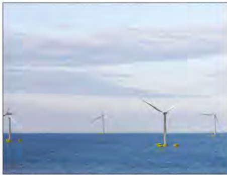
Pentland Demo will support the development of innovative, UK-manufactured floating wind technologies.
