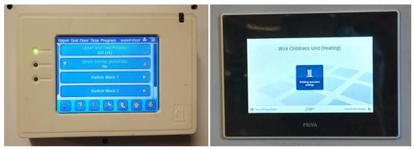
The controller will normally be mounted on the front of plant room control panel and is touch screen operated.
