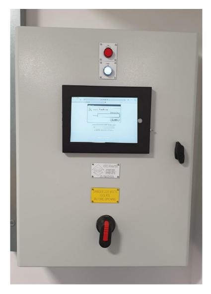
The controller will normally be mounted on the front of plant room control panel and is touch screen operated.
