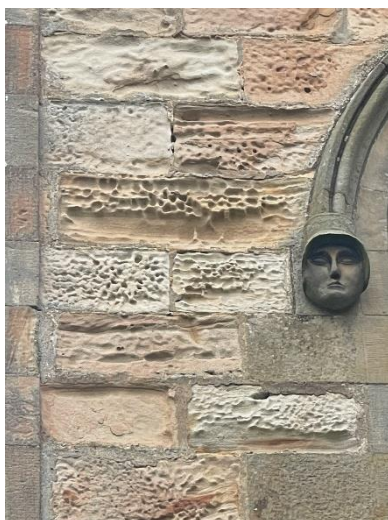
Deteriorating Stonework
