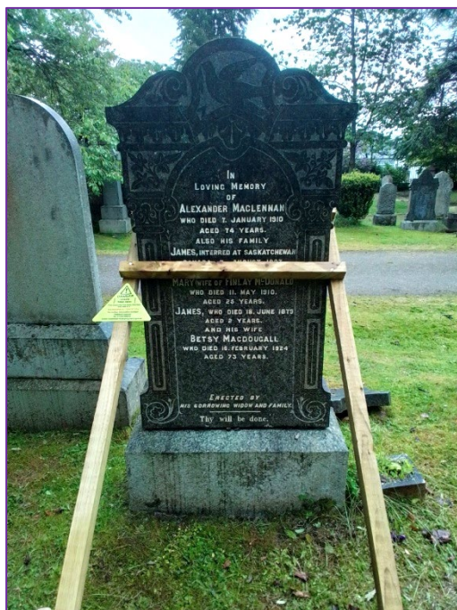
Example of bracing
