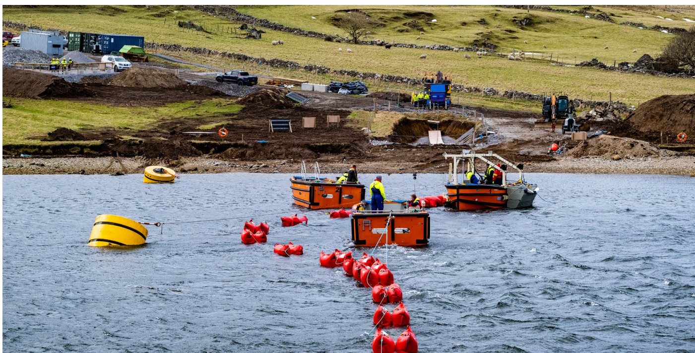
Workers installing a new transmission cable from Shetland to mainland Scotland.
