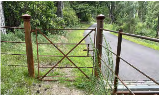
Path gate Untreated steel allowed to rust. Stone posts where available, otherwise cast iron. 1 No.
