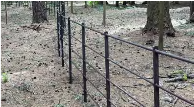
Boundary estate railing to match that at Aldourie Castle Untreated mild steel allowed to rust 880 linear meter
