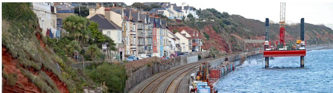
Figure ES9: A repair platform fixes the railway line at Dawlish, Devon, following severe storm damage in 2014. This section of line has had to be repeatedly repaired in the following years, most recently after Storm Ingrid in January 2026. Image credit: Adobe Stock
