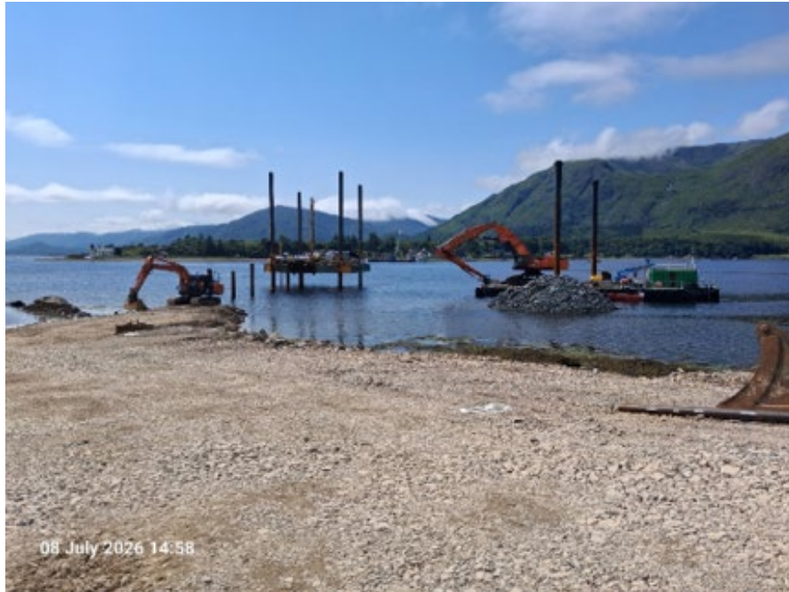
Tubular piling and rock dredging
