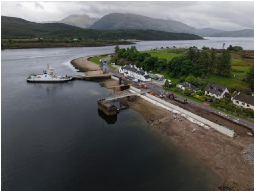
Initial concrete retaining wall construction
