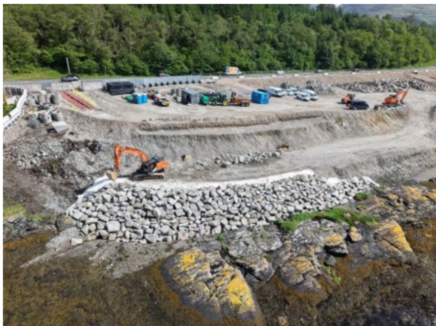
Rock armour placement
