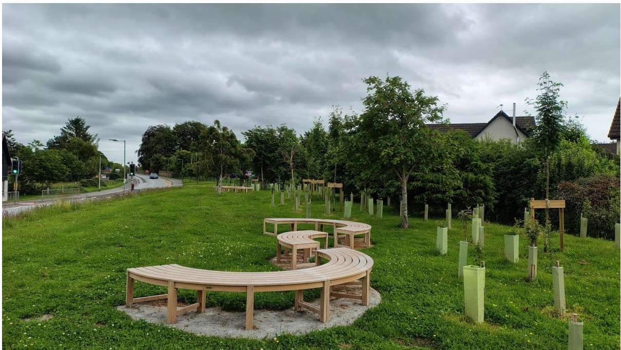
New native species planting and benches next to the school entrance. Footway / crossing improvements and raised table to reduce vehicle speed at the Primary School.
