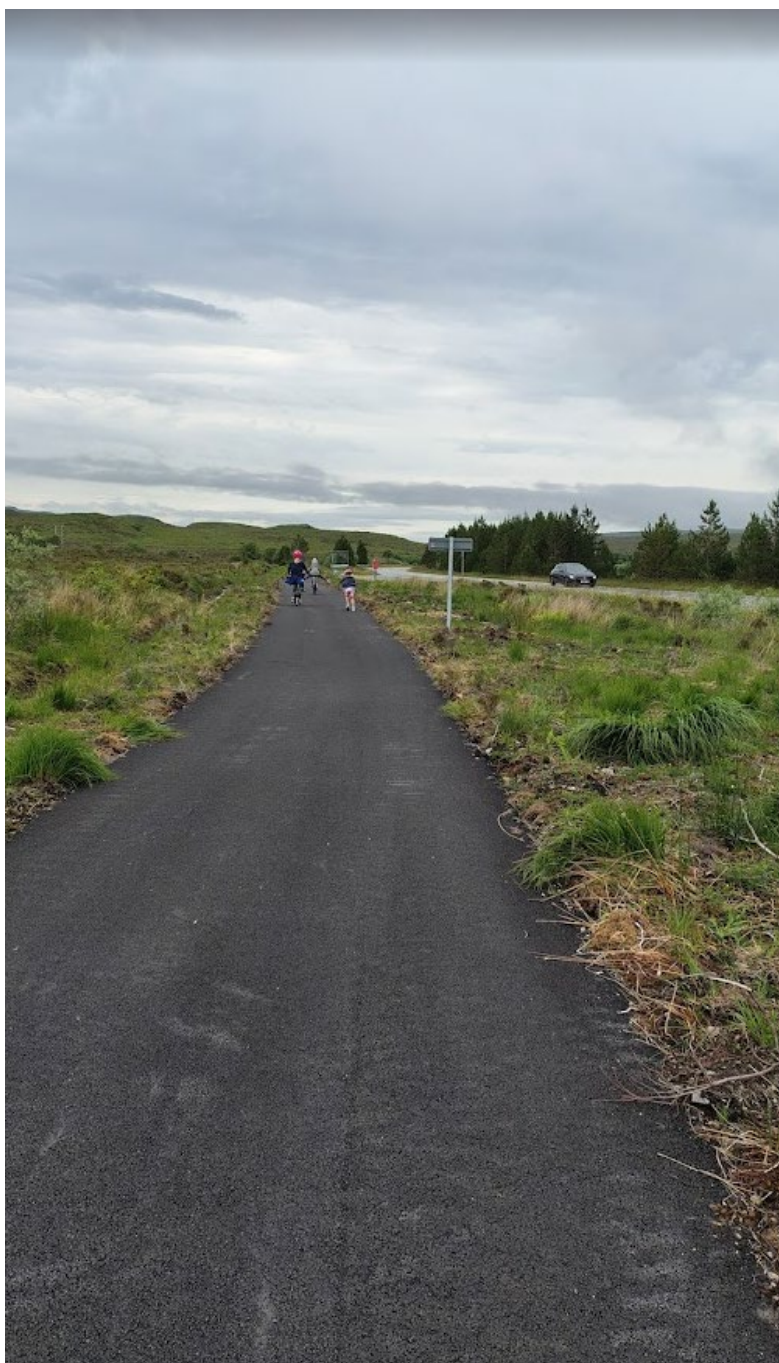
Old Sleat Road, after clearing and scraping
