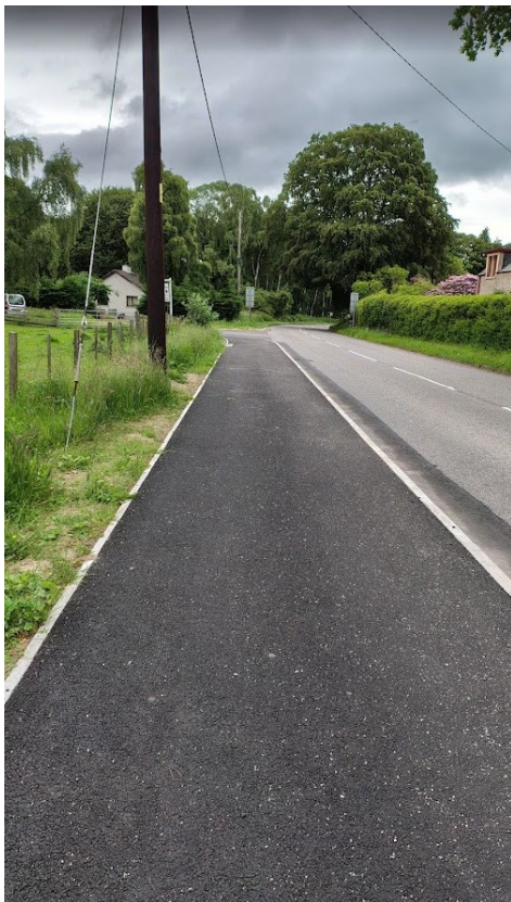
After: new footway in place looking towards Home Farm road end
