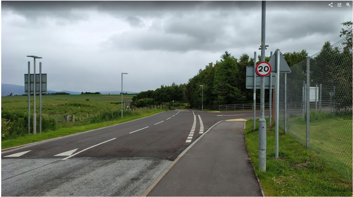
Improved footway to the football pitch and forest walks. Raised table to reduce vehicle speed.
