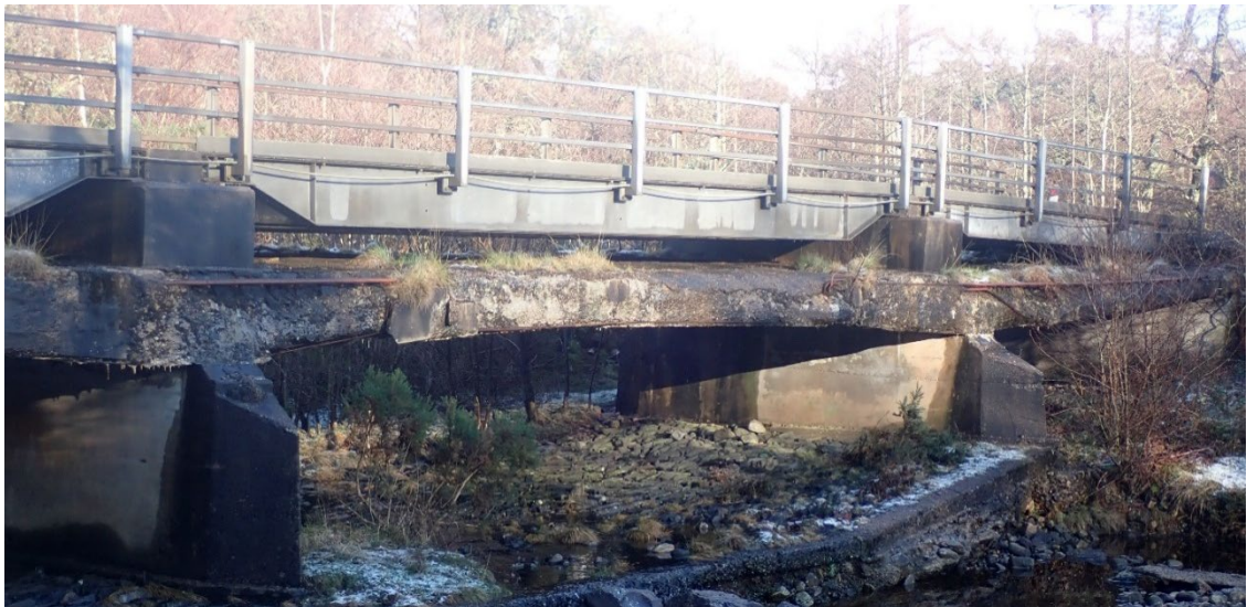
Inverscaddle Overflow bridge (Lochaber)
