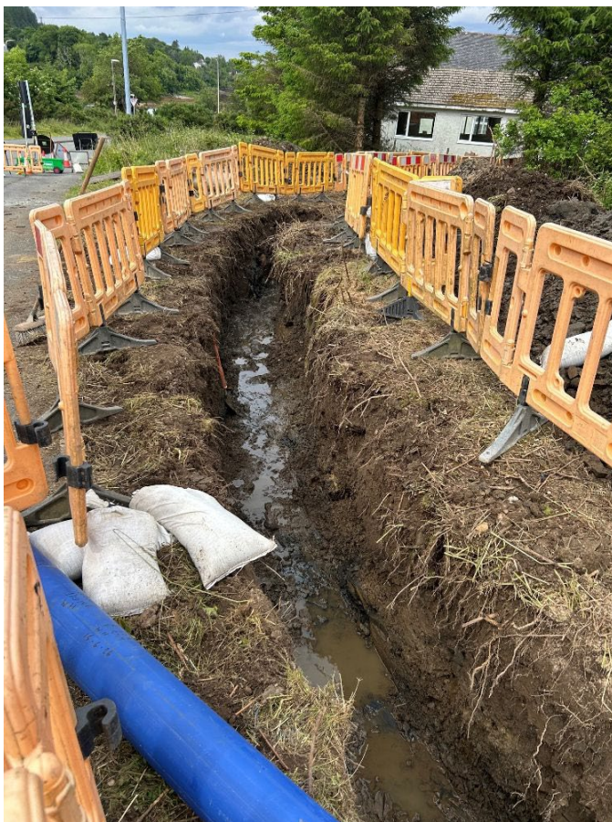
Water main diversion installation
