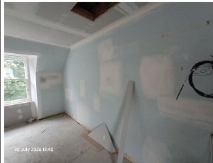
Armoury top floor wall patching progress
