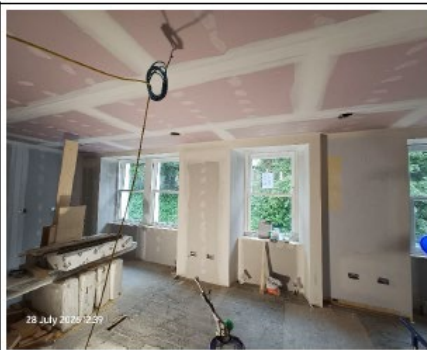
Armoury FF taping progress
