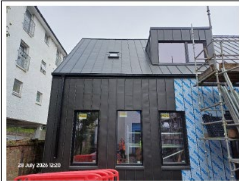
Drill Hall annex scaffold stripped
