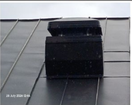
Drill Hall roof venting
