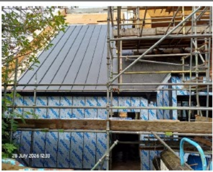
Drill Hall front elevation zinc progress
