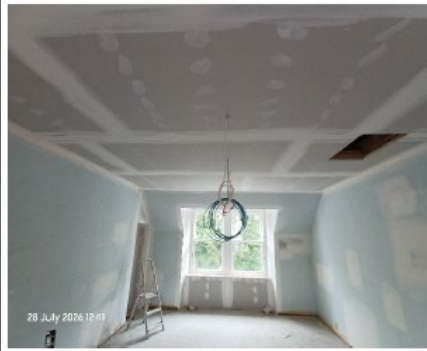
Armoury top floor taping progress
