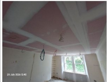
Armoury FF taping progress
