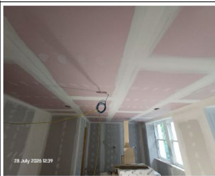
Armoury FF taping progress ceilings and walls
