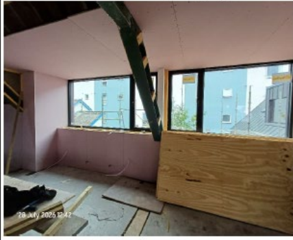
Drill Hall rear elevation dormer internal progress
