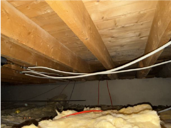
Photograph 08 – First Floor Joists and Beam
