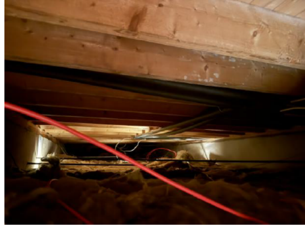
Photograph 09 – First Floor Joists and Ceiling
