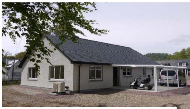
CHT Adapted Built home, Invergarry.
