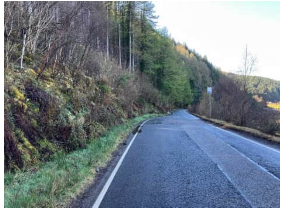
Photo at End Chainage (looking east)
