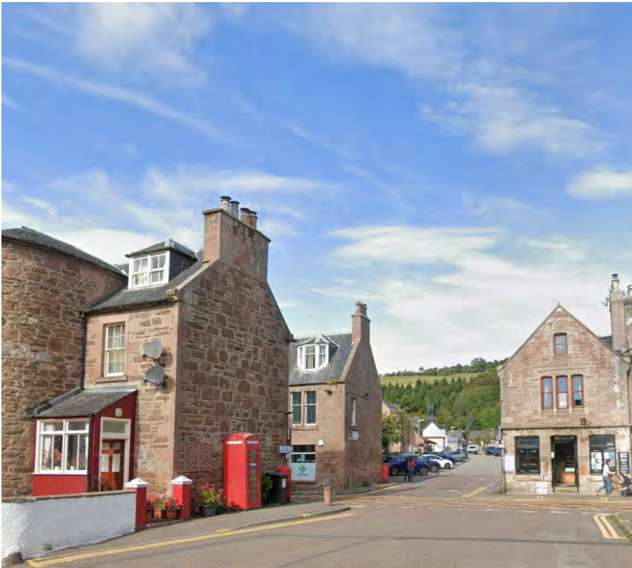
Fortrose village - Red sandstone, cladding, window frames and gate posts.
