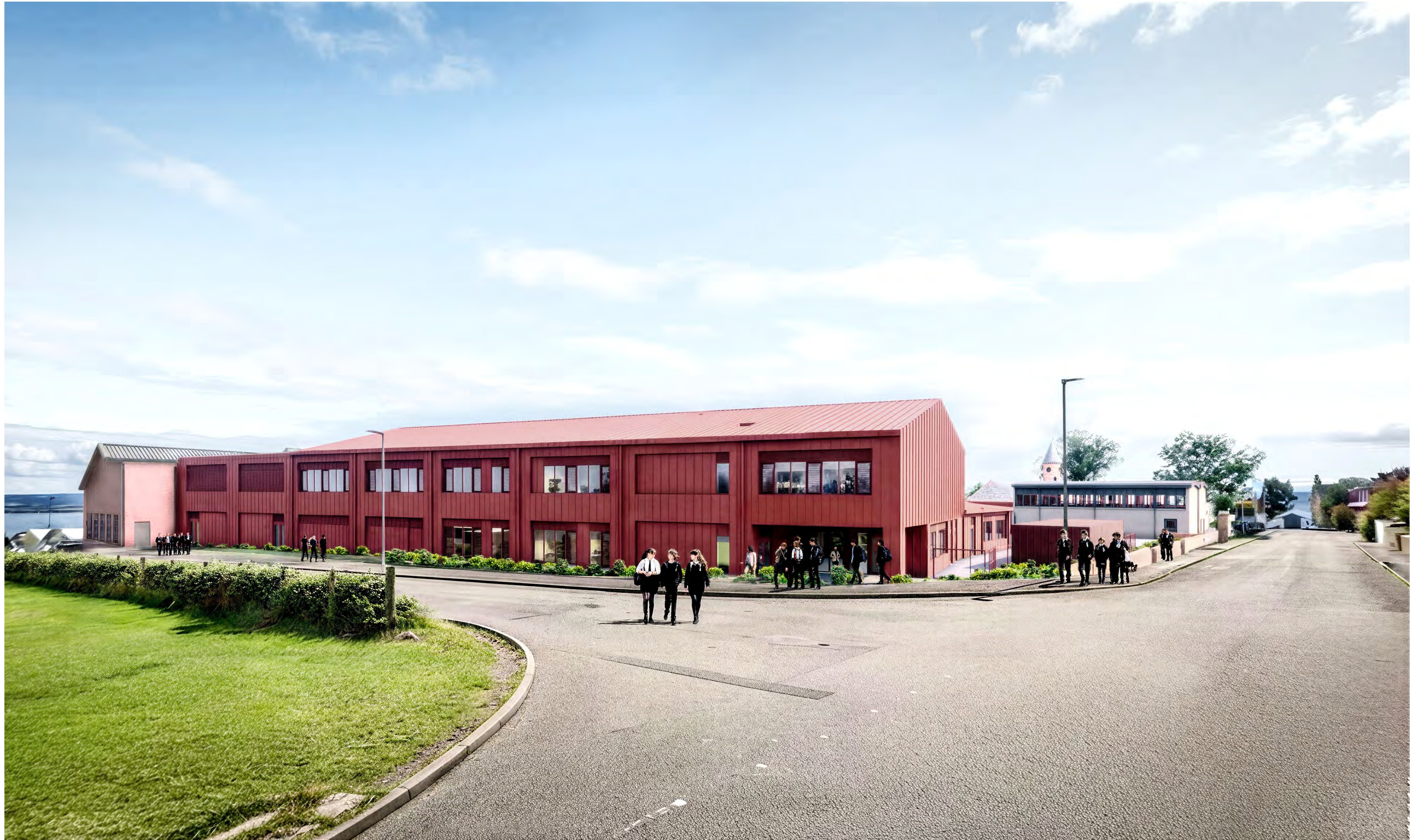
Newbuild Teaching Block - View from Deans Road
