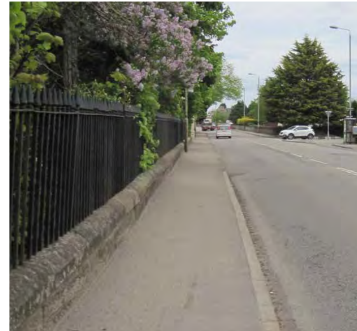
Simple, appropriate, easily repaired paving.
