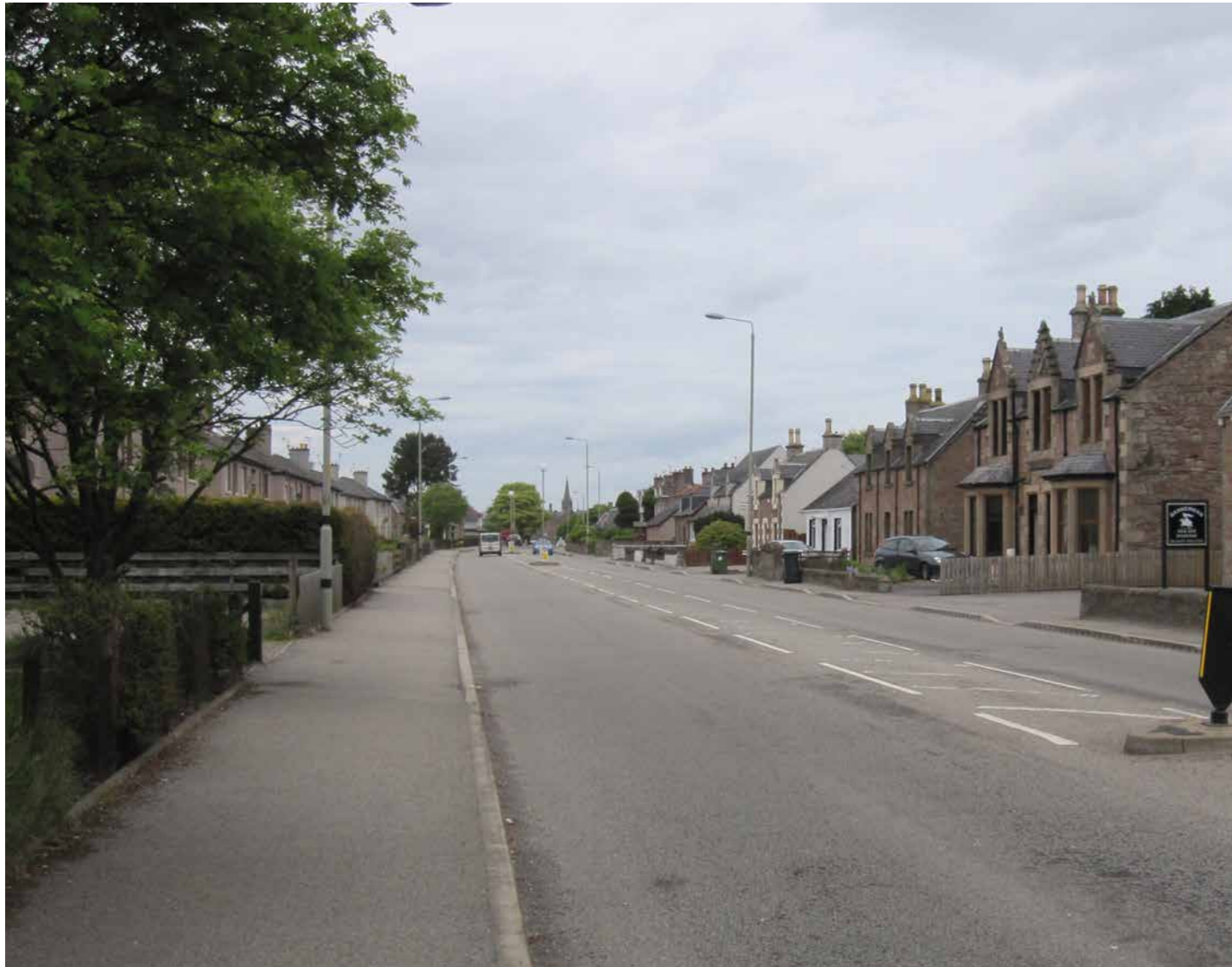
1:4.5 enclosure - a main suburban street, generous set-back of housing on the right leads to a slightly open character. Loss of garden walls to allow frontage parking starting to degrade the character of the street.
