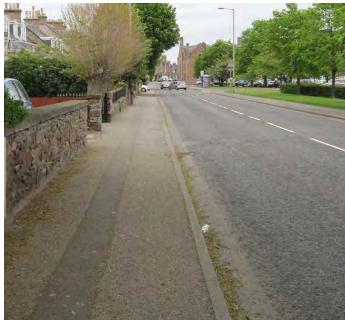
'Skinny' kerbs: traditionally used in 'normal streets'.
