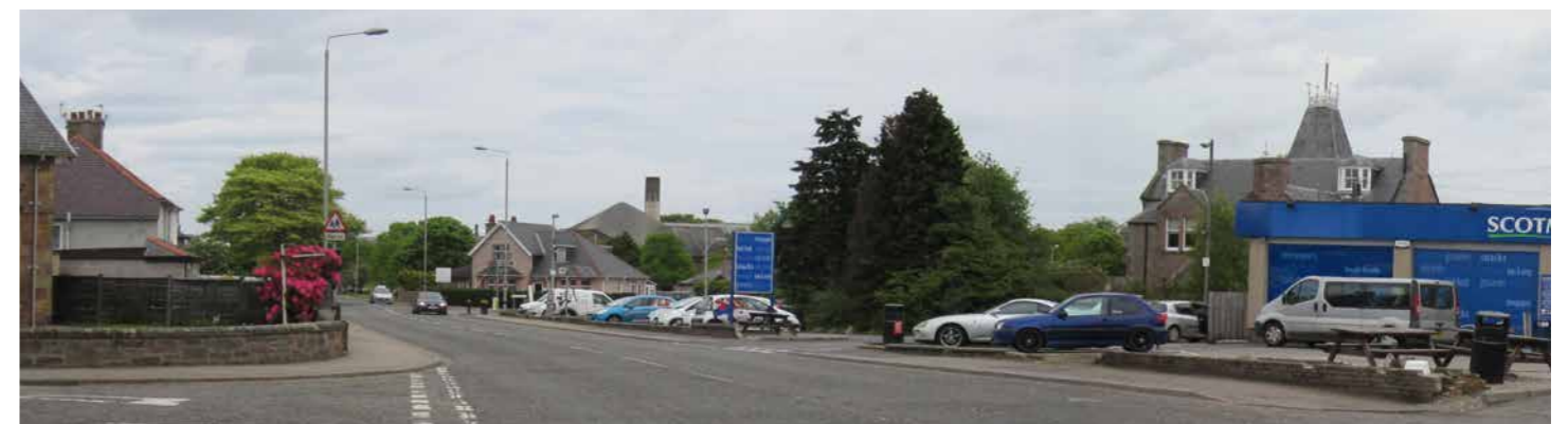
Open frontage and inappropriate building line detract from the character of the townscape.
